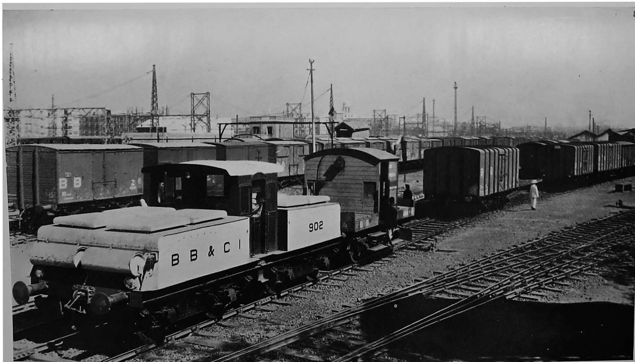
Battery Locomotive in use at Carnac Bunder.
