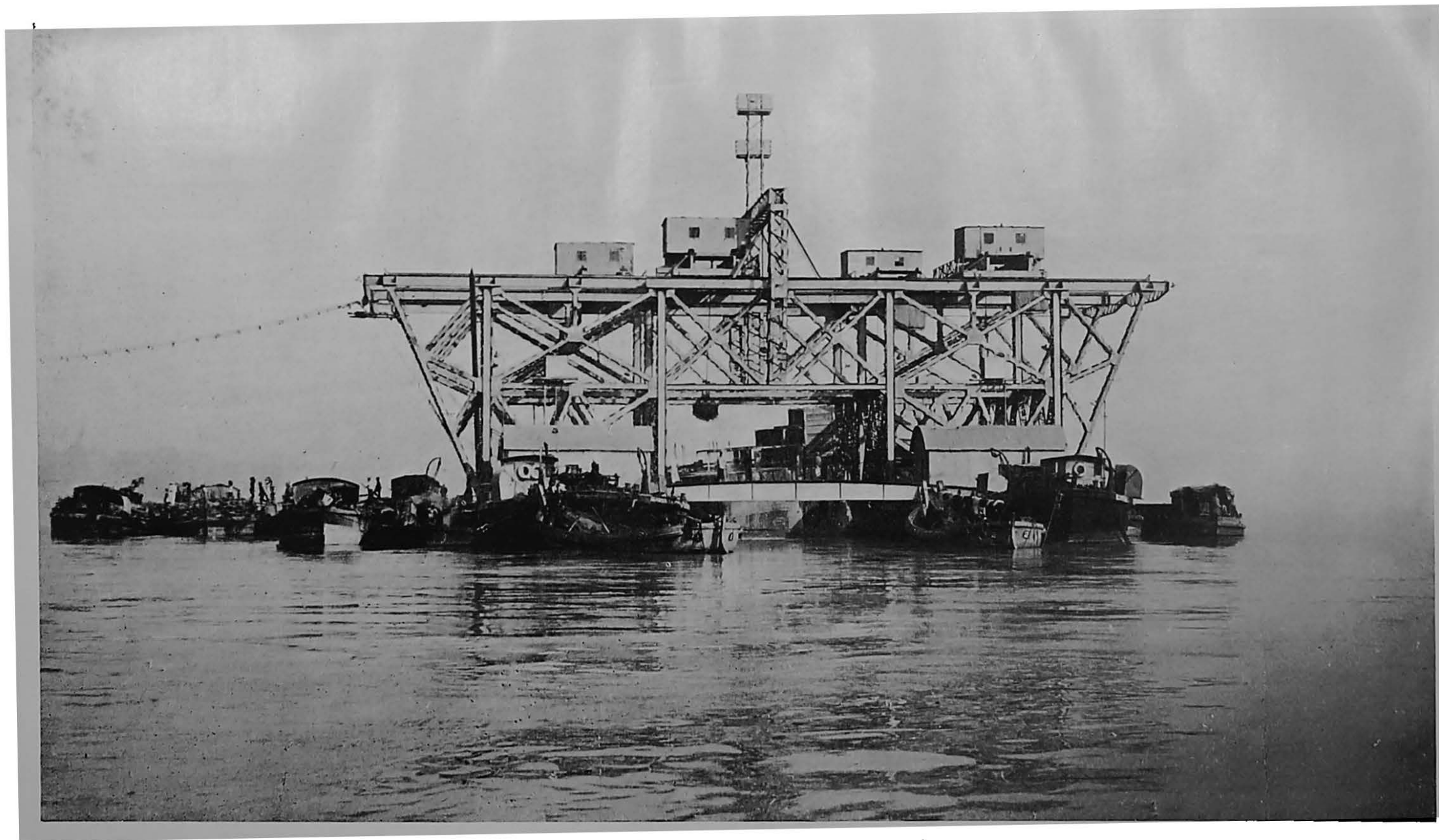
Bally Bridge—Dredging at No. 3 Pier (12th January 1929).
