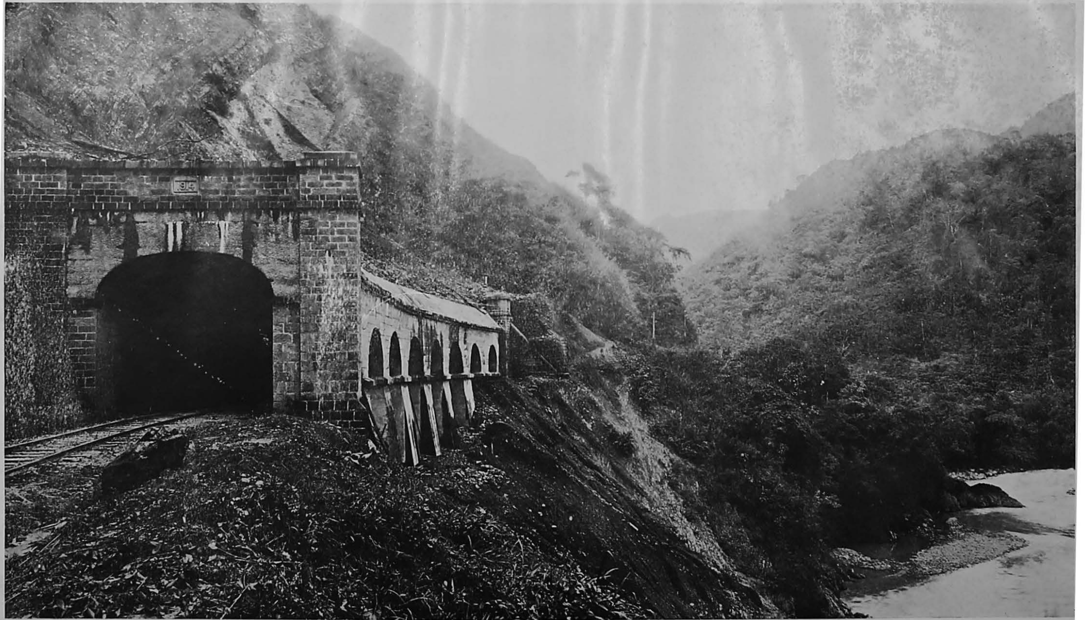
Covered way carried on Viaduct at Chamartola.
