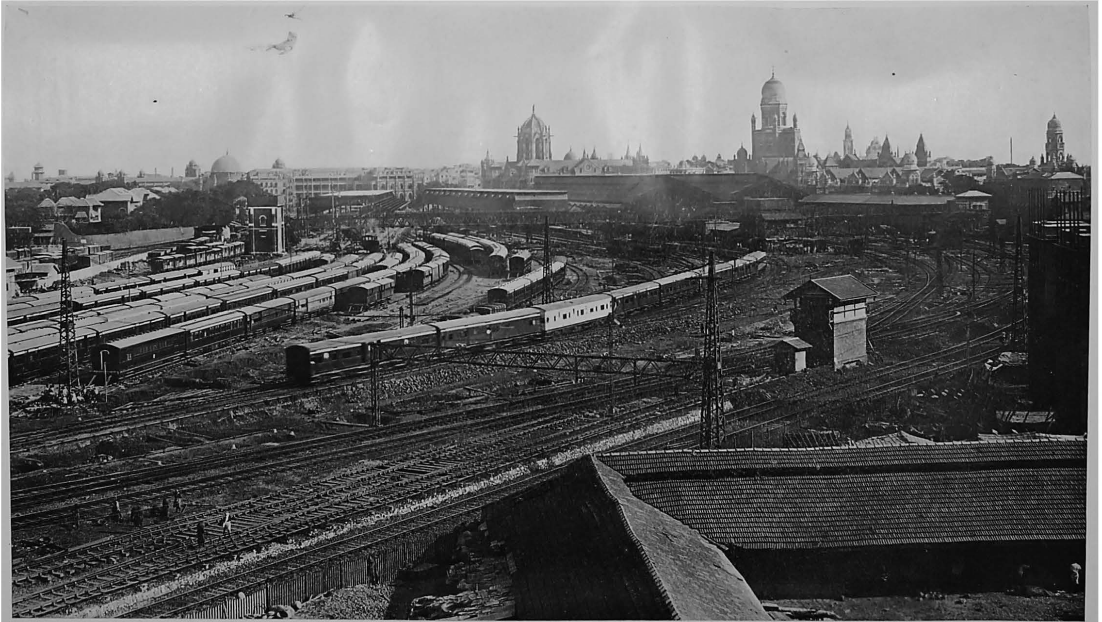
Remodelling of Victoria Terminus Yard—"Work in Progress."
