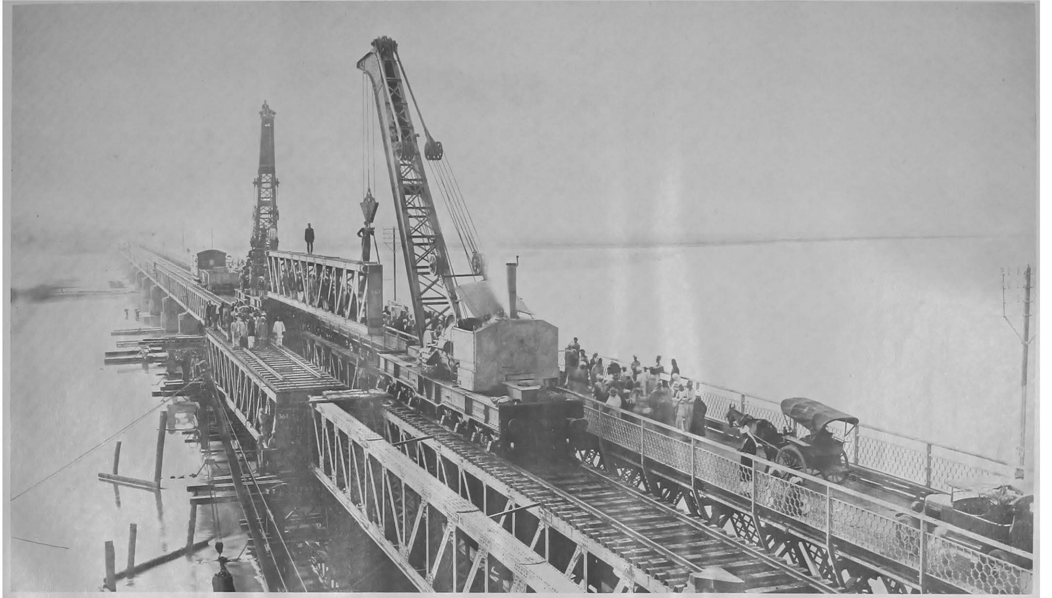
Regirding of Jhelum Bridge
