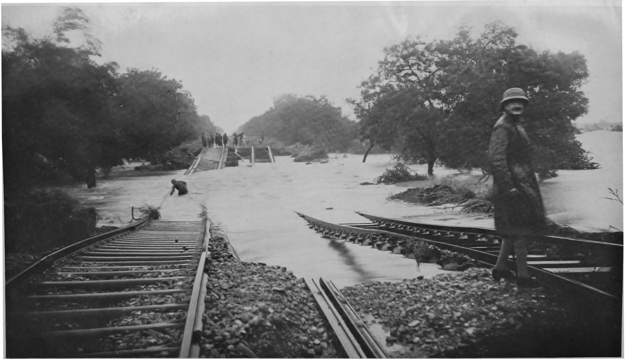
Breaches in Main Line near Itola, July 1927
