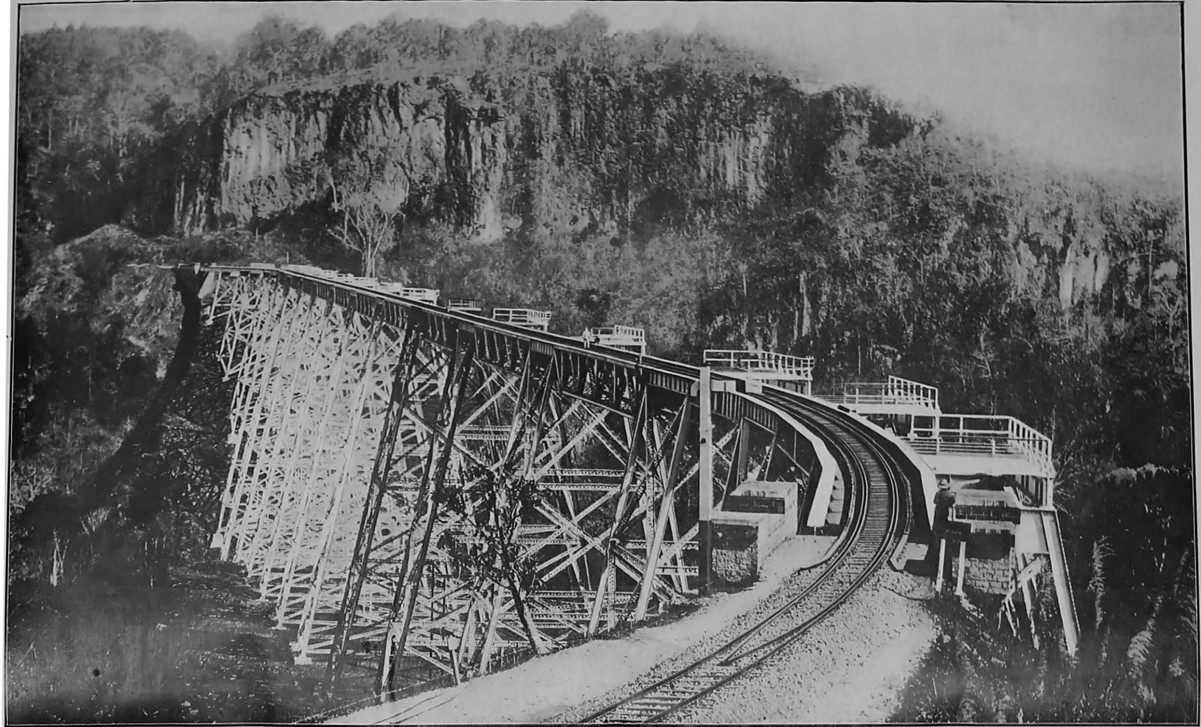
Gobleib Viaduct —A work of great engineering interest on the Burma Railways constructed over a deep gorge on the Chungzoune river which disappears in a natural tunnel 500 feet below the
