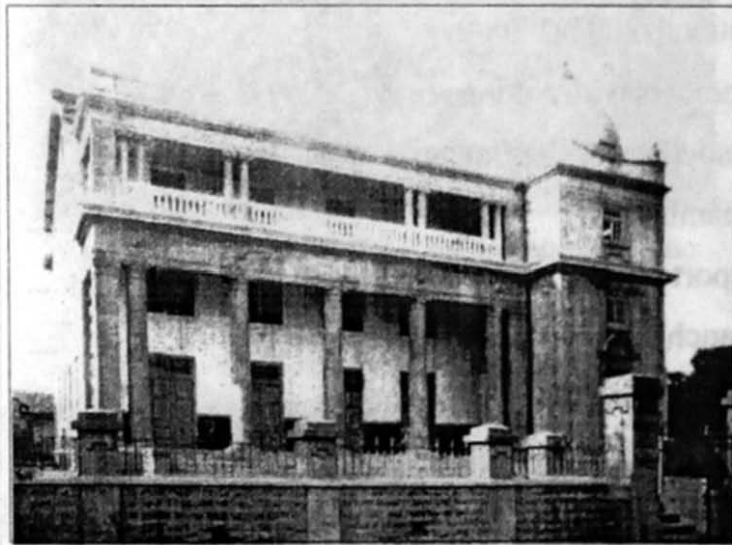
Gokhale Hall Building Situated at Laxmi Road, Pune
