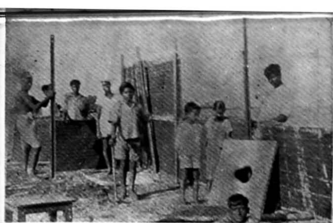
The borehole latrine Construction by boys.
