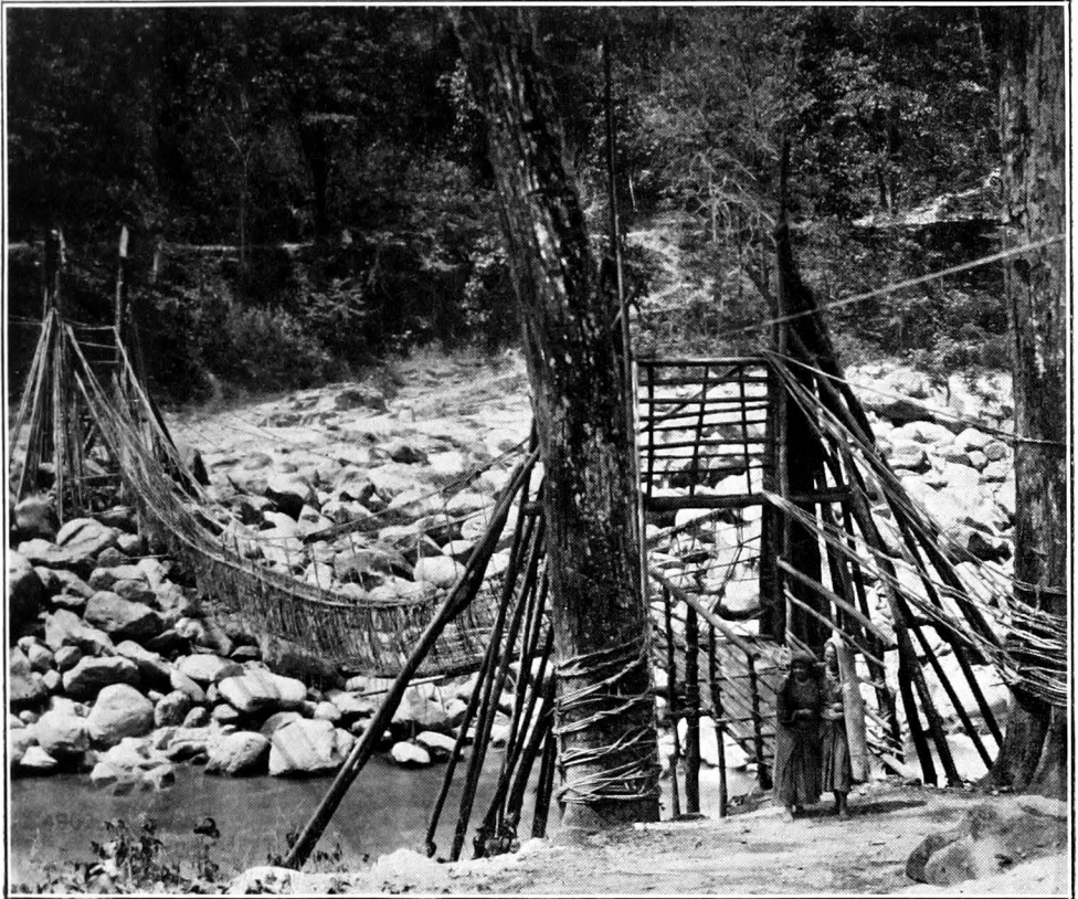
CANE BRIDGE ON THE RUNGIT RIVER.
