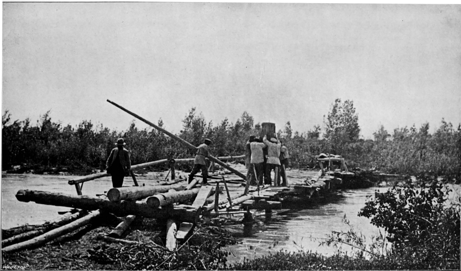
A BROKEN BRIDGE ON THE POST-ROAD.
