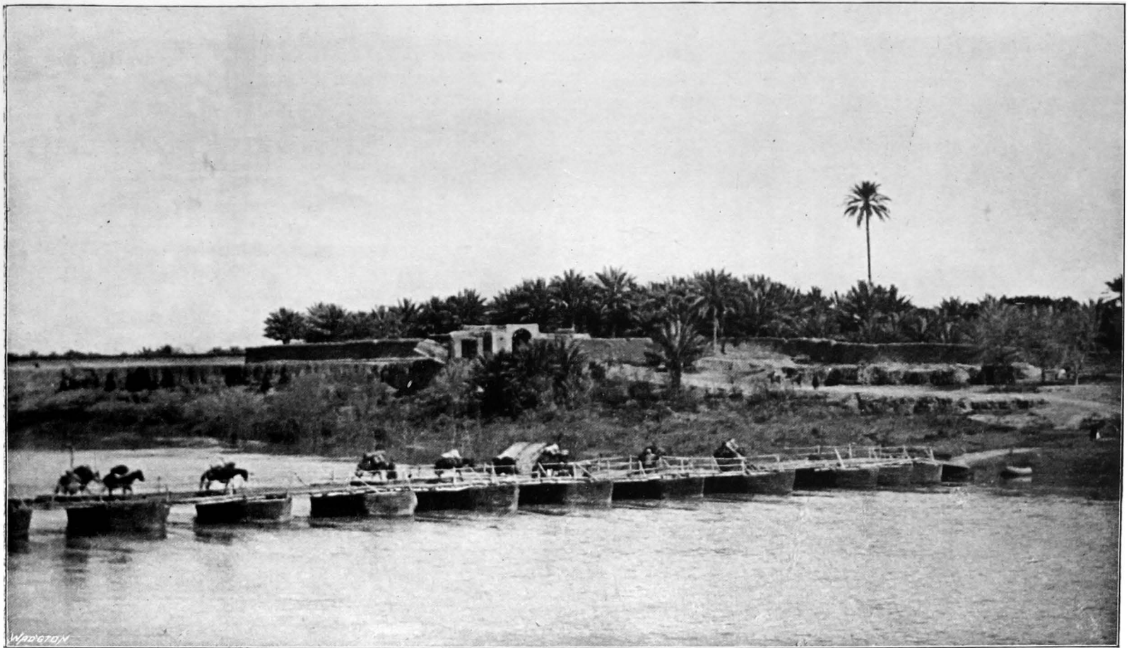
BRIDGE OVER THE DIALA.
