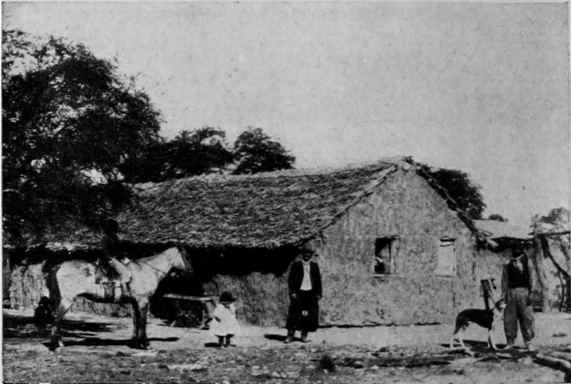
FIG. 370.—A sod house on the Argentine Pampa. (Photograph by H. G. Olds.)
