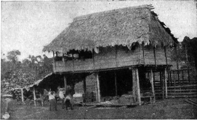
FIG. 368.—A native house in the tropical rainforest of Ecuador. The living quarters are elevated above the ground in order to protect against floods and animals and to give better under-ventilation. ( Rau Art Studios. )
