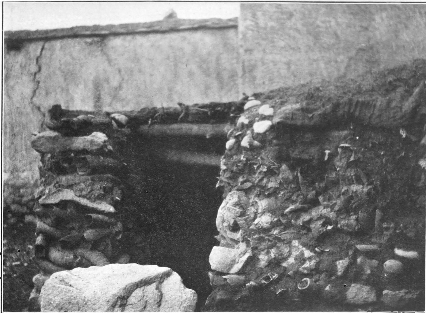
A typical mud and horn hut of a Ragyaba. It is about four feet high.
