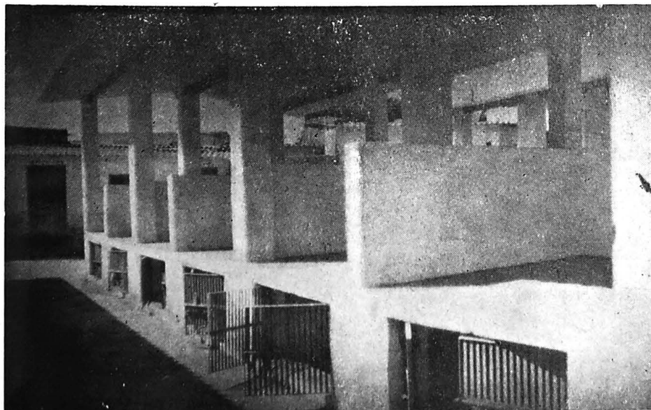
PHOTOGRAPH No. 16 Newly constructed Vegetable Market, Camp No. 4
