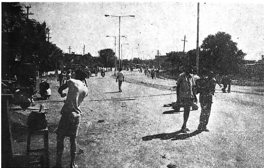
PHOTOGRAPH No. 15 A good road in camp No. 5, Southern part of Ulhasnagar.
