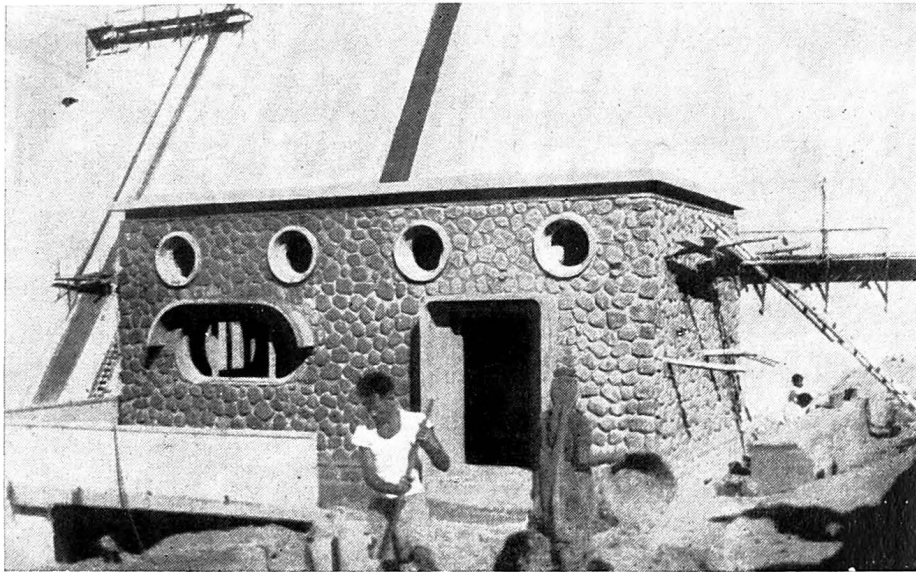
Permanent Pump House at Vaitarna
