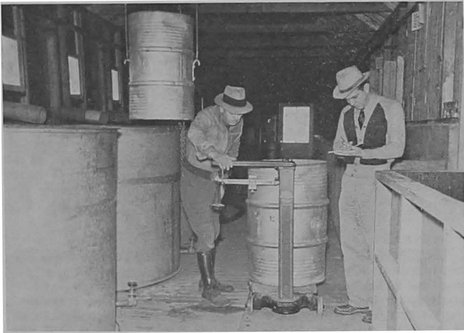
FIGURE 4. INTERIOR OF THE BUILDING SHOWN IN FIGURE 3
