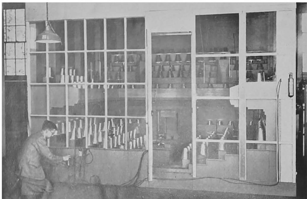
*Above* : The quarter-scale model used to investigate the behaviour of the novel system of ventilation now installed in the Debating Chamber of the new House of Commons. *Below* : In this supersonic wind tunnel a model of a German V2 was tested before the rocket attack was launched against London
