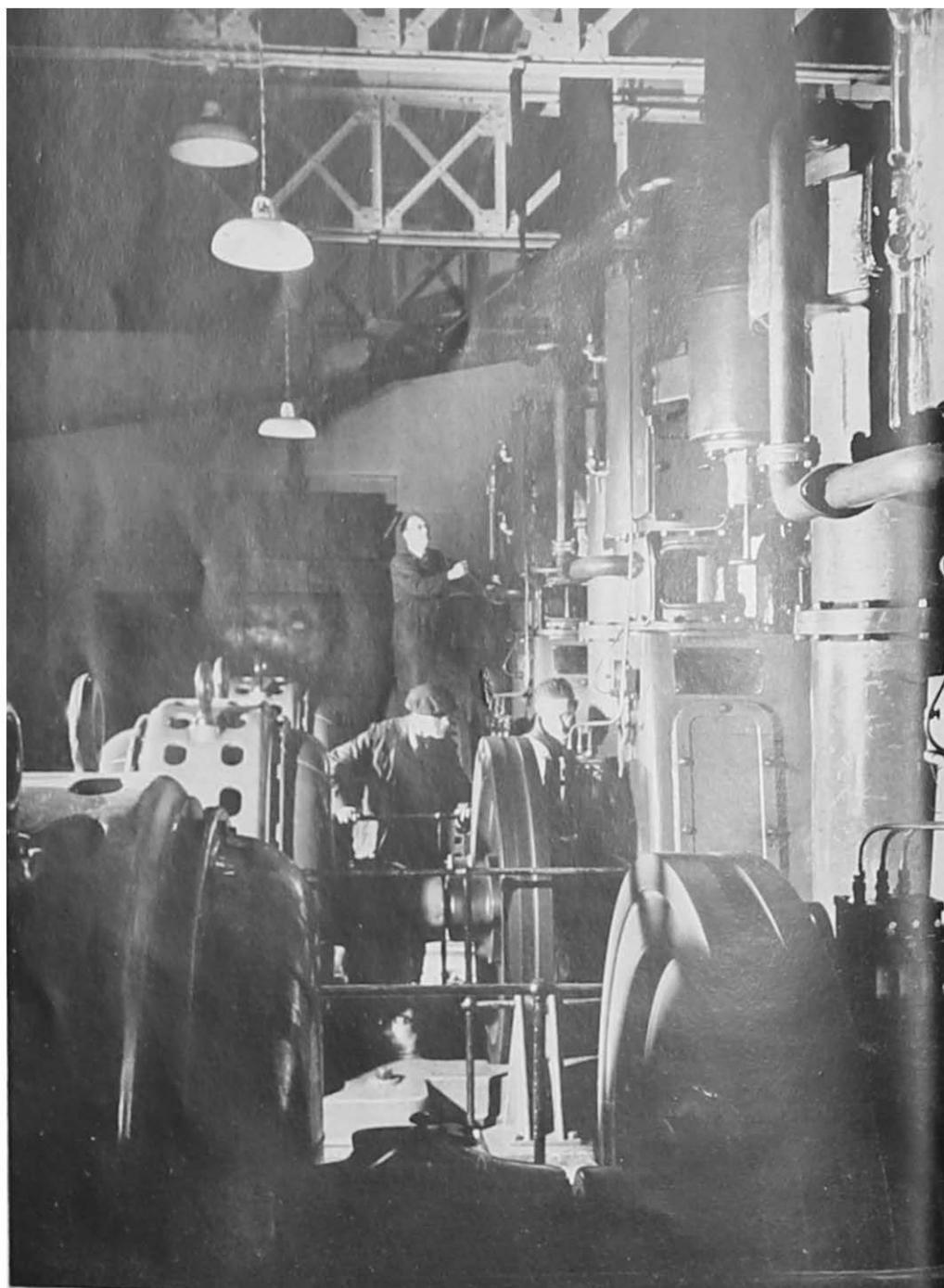
Three heavy duty compressors can produce a pressure of 25 atmospheres in one hour in the compressed air tunnel, providing model testing conditions equivalent to those of full-scale flight
