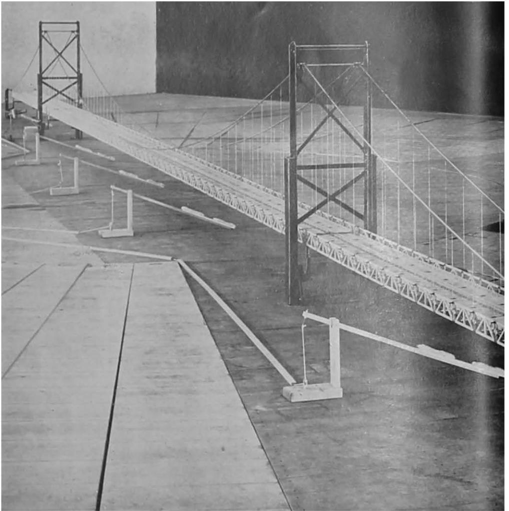
The 50-ft model of the proposed suspension bridge over the River Severn is tested in a specially constructed wind tunnel to investigate the effects of various winds on the structure. The devices to be seen on the left of the bridge are arresters for controlling the oscillations of the model
