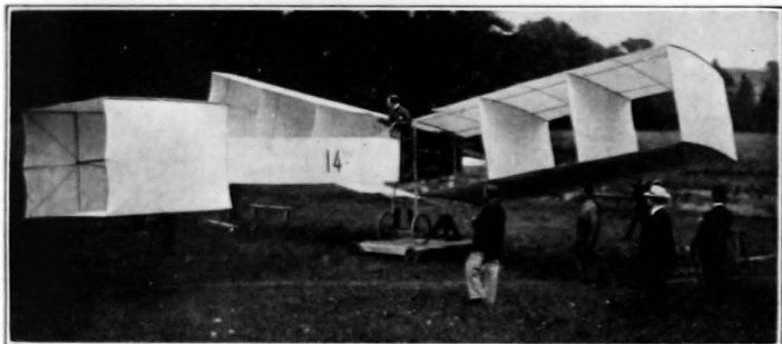
THE SANTOS DUMONT CANARD OR TAIL FIRST AEROPLANE. This aircraft was fitted with side curtains to provide lateral as well as directional stability. The Aircraft flew successfully.
