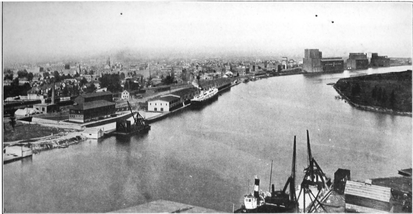
THE TWIN CITIES OF PORT ARTHUR AND FORT WILLIAM AT THE HEAD OF THE GREAT LAKES, THE CHIEF OUTLET FOR THE GRAIN TRAFFIC OF THE CANADIAN WEST.
