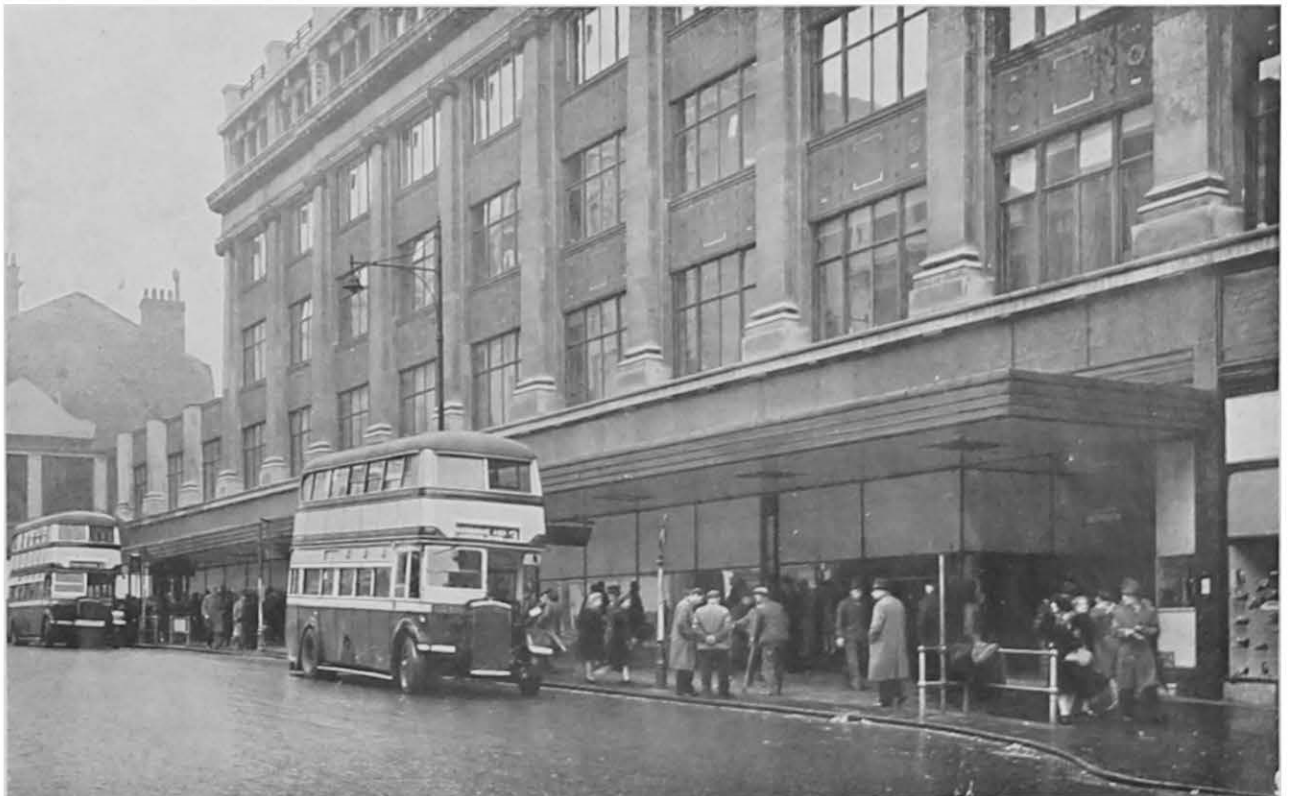
PLATE 2. BUS QUEUE BARRIERS BELOW CANOPY—BIRMINGHAM.
