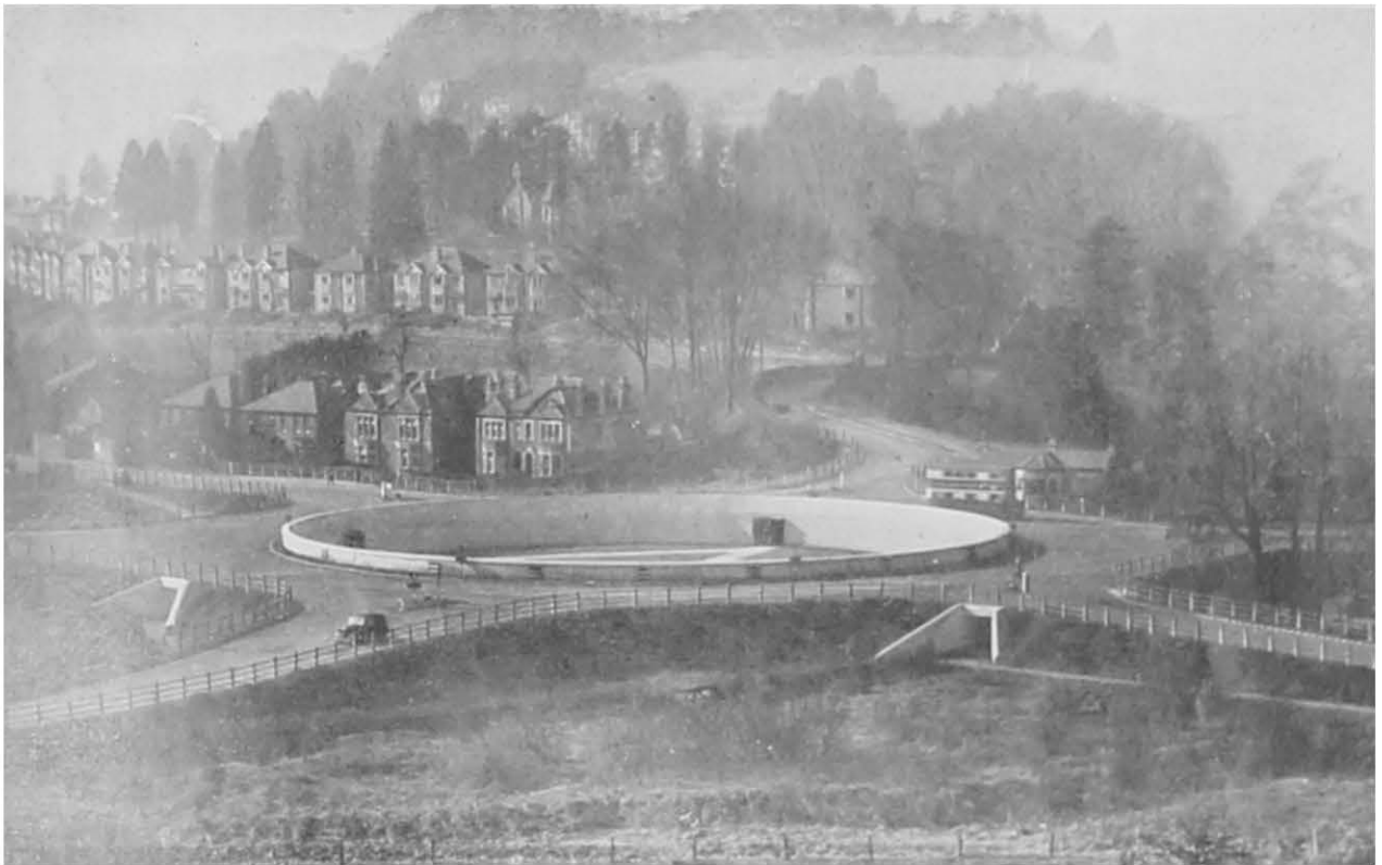
PLATE 23. TWO-LEVEL ROUNDABOUT WITH PEDESTRIAN SUBWAYS—CATERHAM, SURREY.
