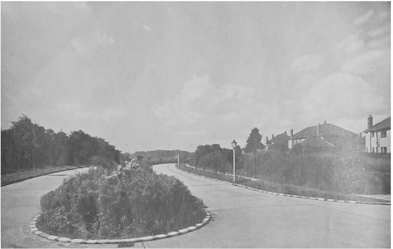
PLATE 17. DEVELOPMENT, HAVING NO ACCESS TO RING ROAD, SCREENED BY SHRUBS AND TREES—LEEDS.
