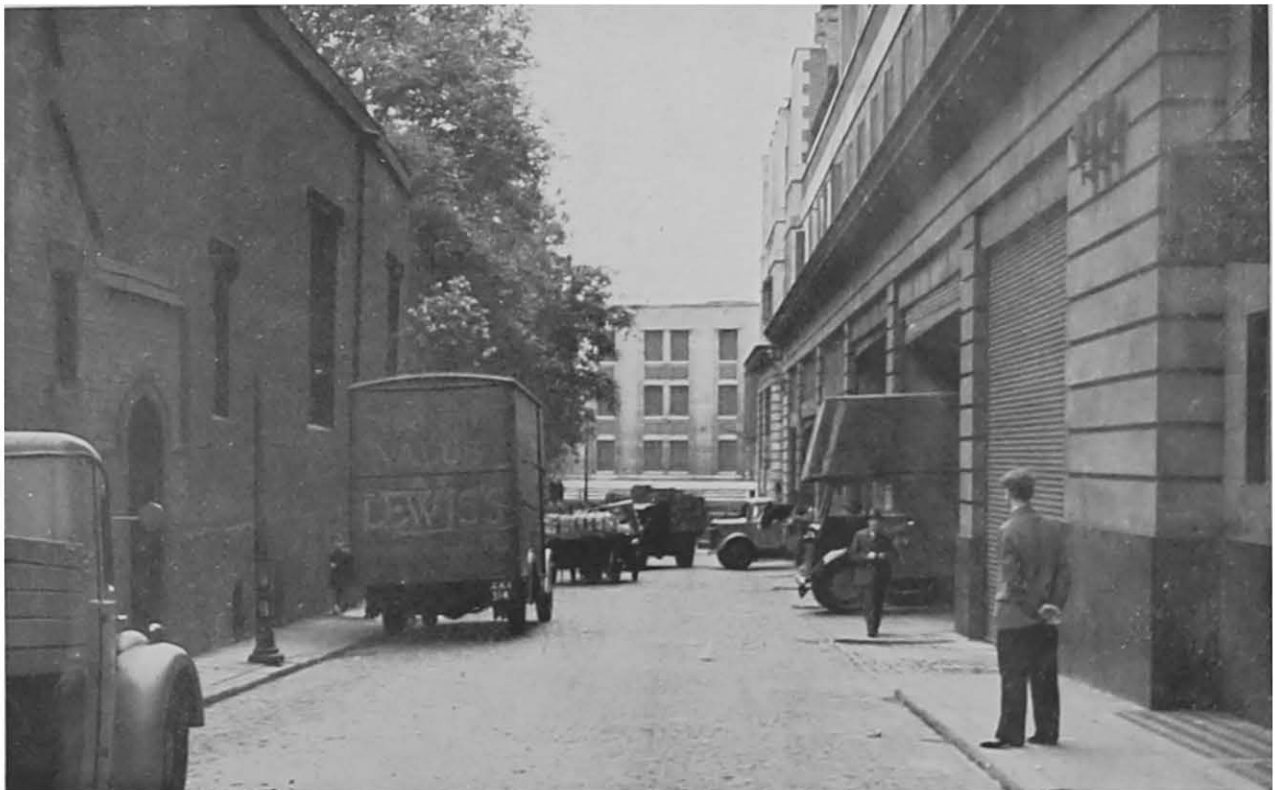
PLATE 6. BACK ACCESS LANE WITH LOADING BAYS IN BUILDING—LEEDS.
