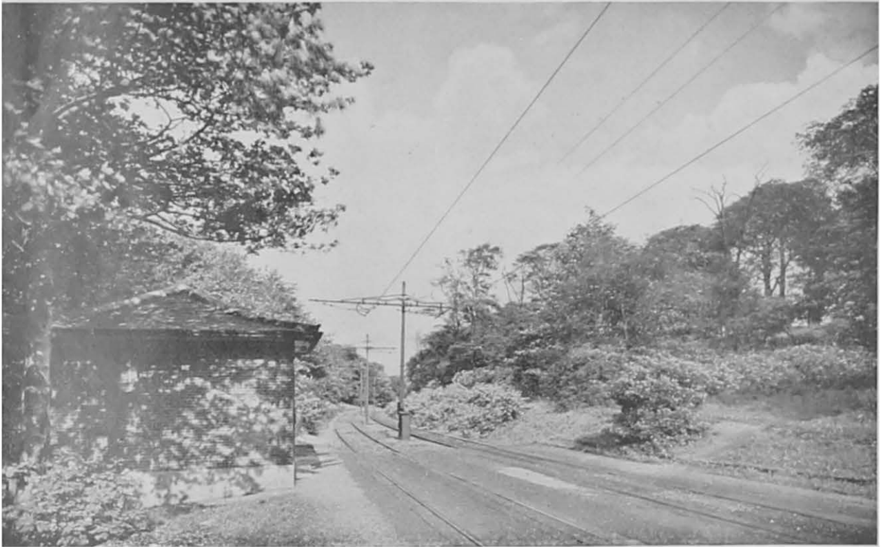
PLATE 19. TRAMWAY IN RESERVATION OFF THE HIGHWAY—LEEDS.
