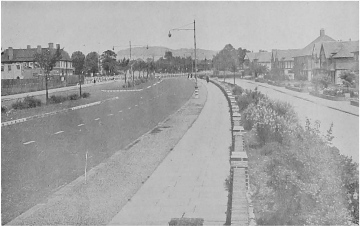
PLATE 21. SERVICE ROAD SEPARATED FROM DUAL CARRIAGEWAY ROAD BY SHRUBBERY AND LOW WALL—WOOLWICH,
