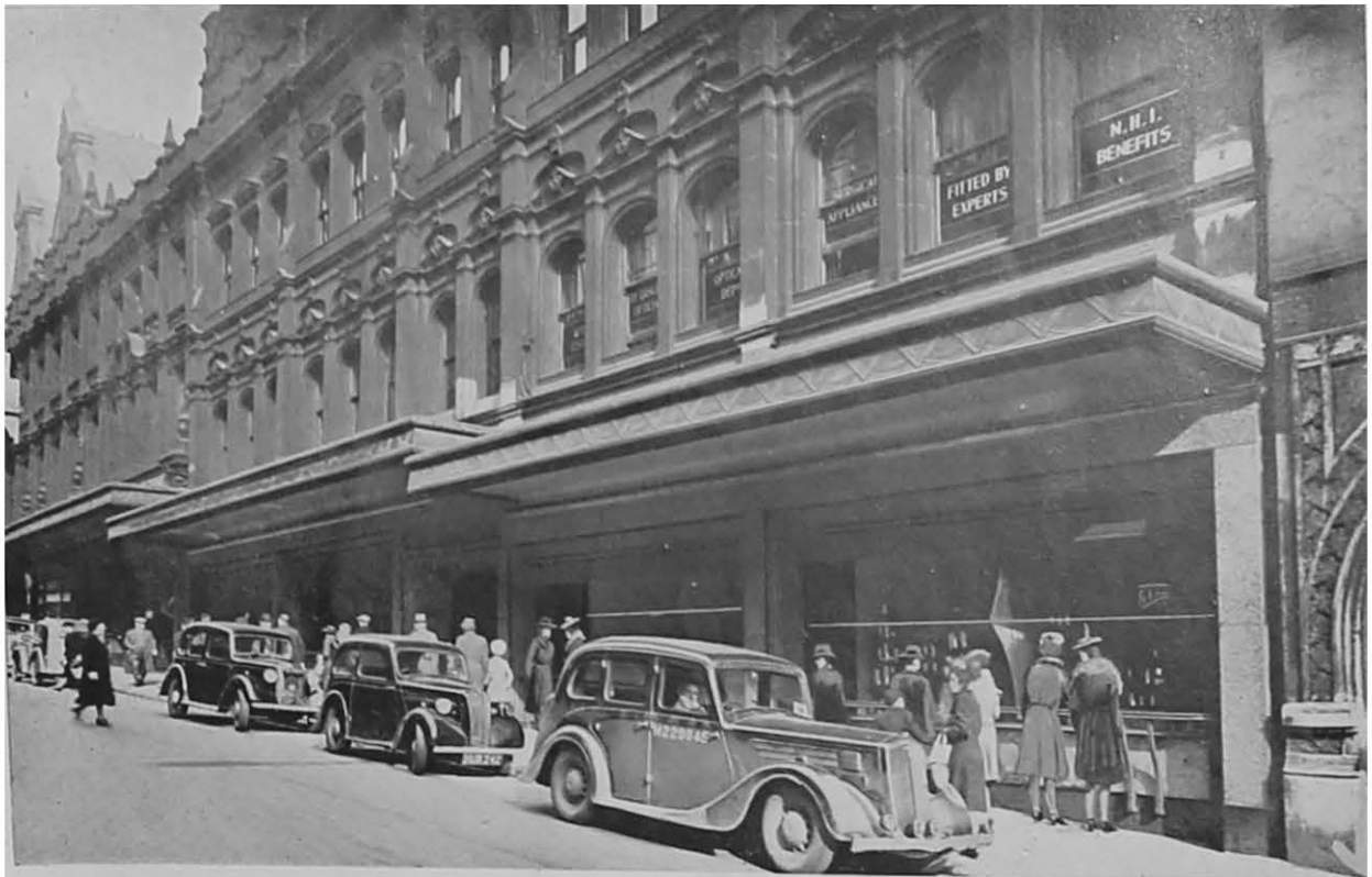
PLATE 8. CANOPIES CANTILEVERED FROM BUILDINGS—LEEDS.
