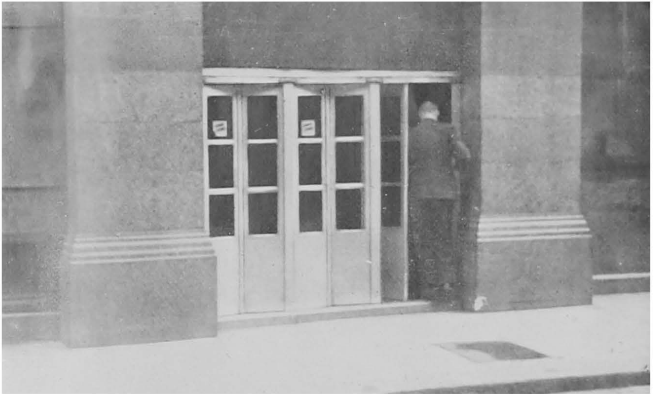
PLATE 34. TELEPHONE BOXES BUILT INTO WALL OF BUILDING—LONDON.
