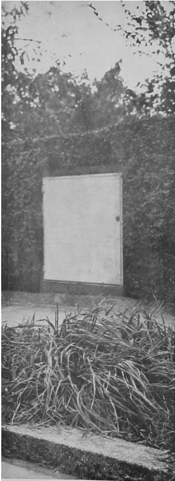
PLATE 32. . ELECTRICITY BOX SITED IN HEDGE—FINCHLEY.
