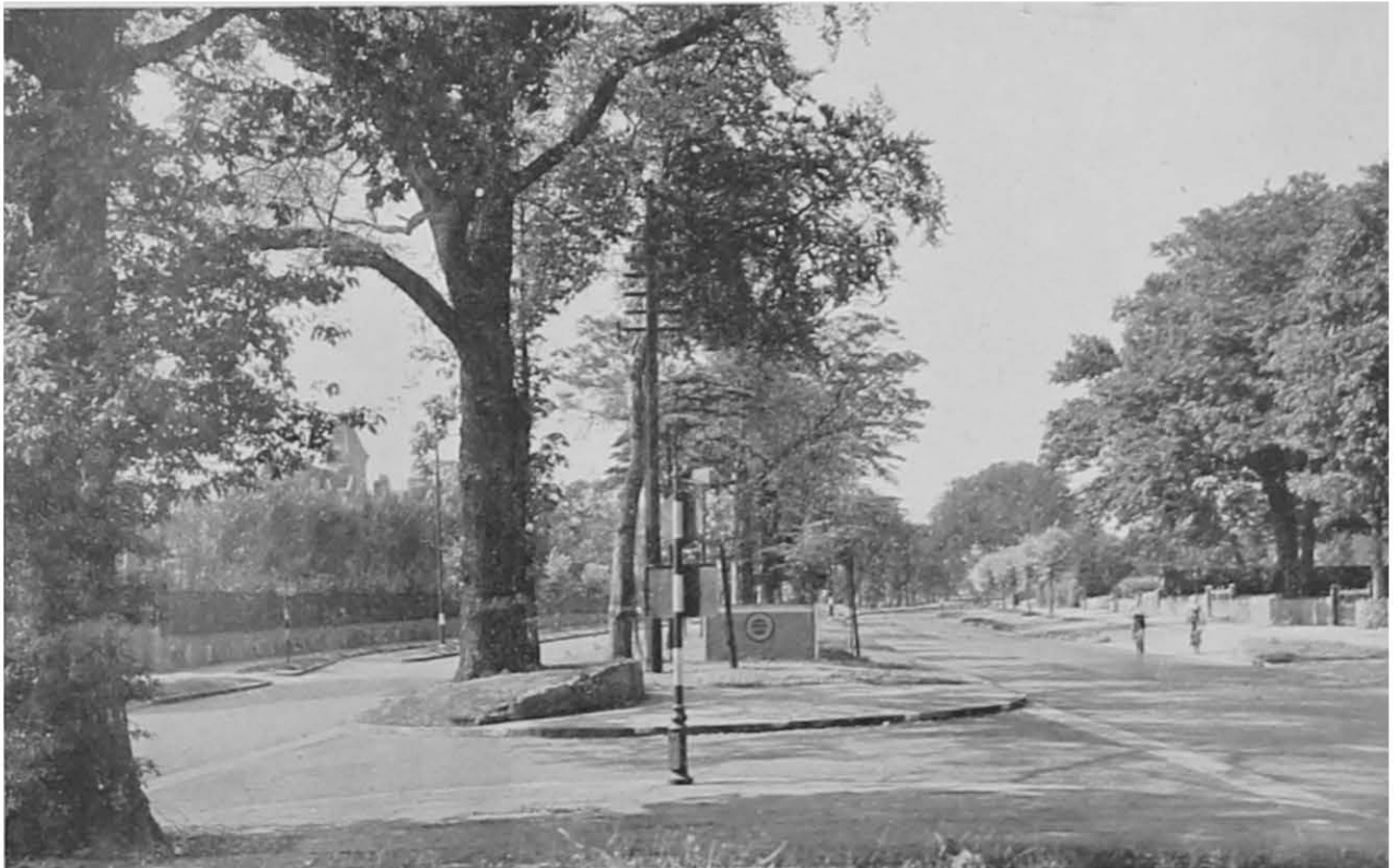
PLATE 20. DUAL CARRIAGEWAY ROAD WITH CYCLE TRACKS—BIRMINGHAM.
