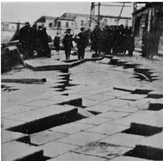
A. MESSINA EARTHQUAKE. Subsidence of quay at Messina (Baratta).
