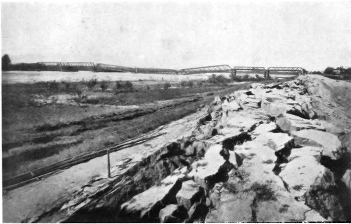
B. MINO-OWARI EARTHQUAKE. Fissures in embankment of R. Nagara and damaged railway bridge (Milne and Burton).
