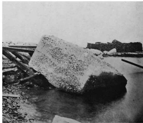
B. MESSINA EARTHQUAKE. Transport of block of concrete by seawave (Omori).
