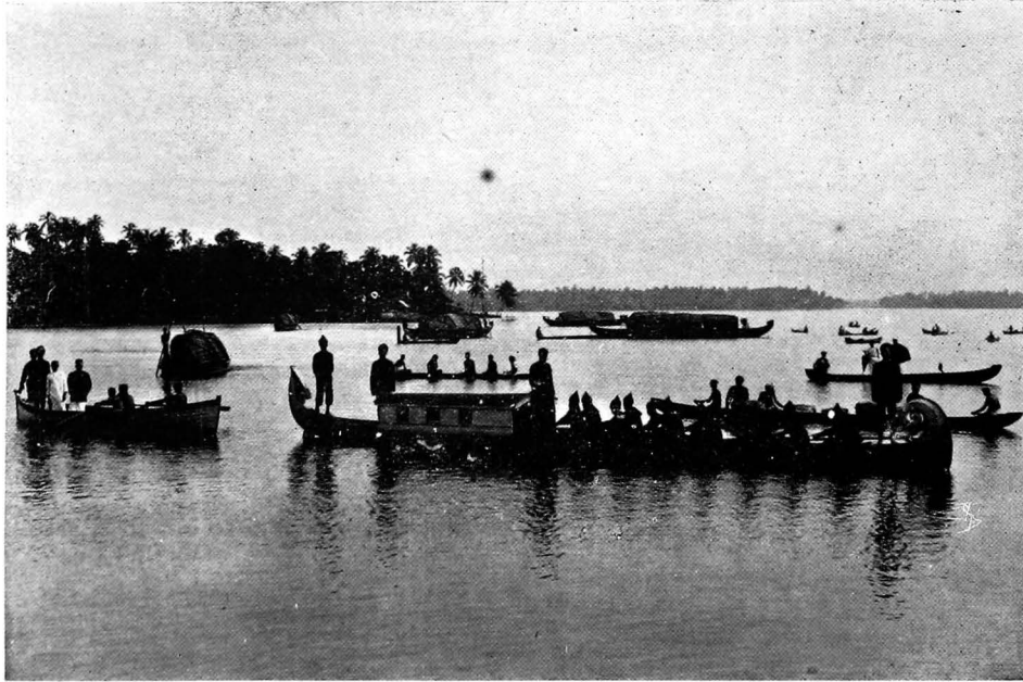
A CANAL VIEW.
