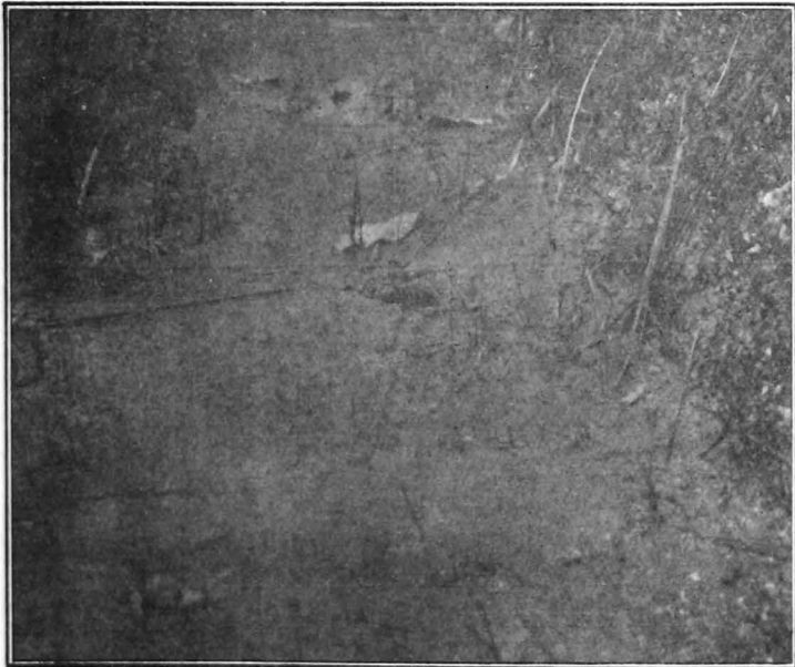
Showing the effect of digging a hole through the impervious surface layer of clay deposited in the drain from the bank.
