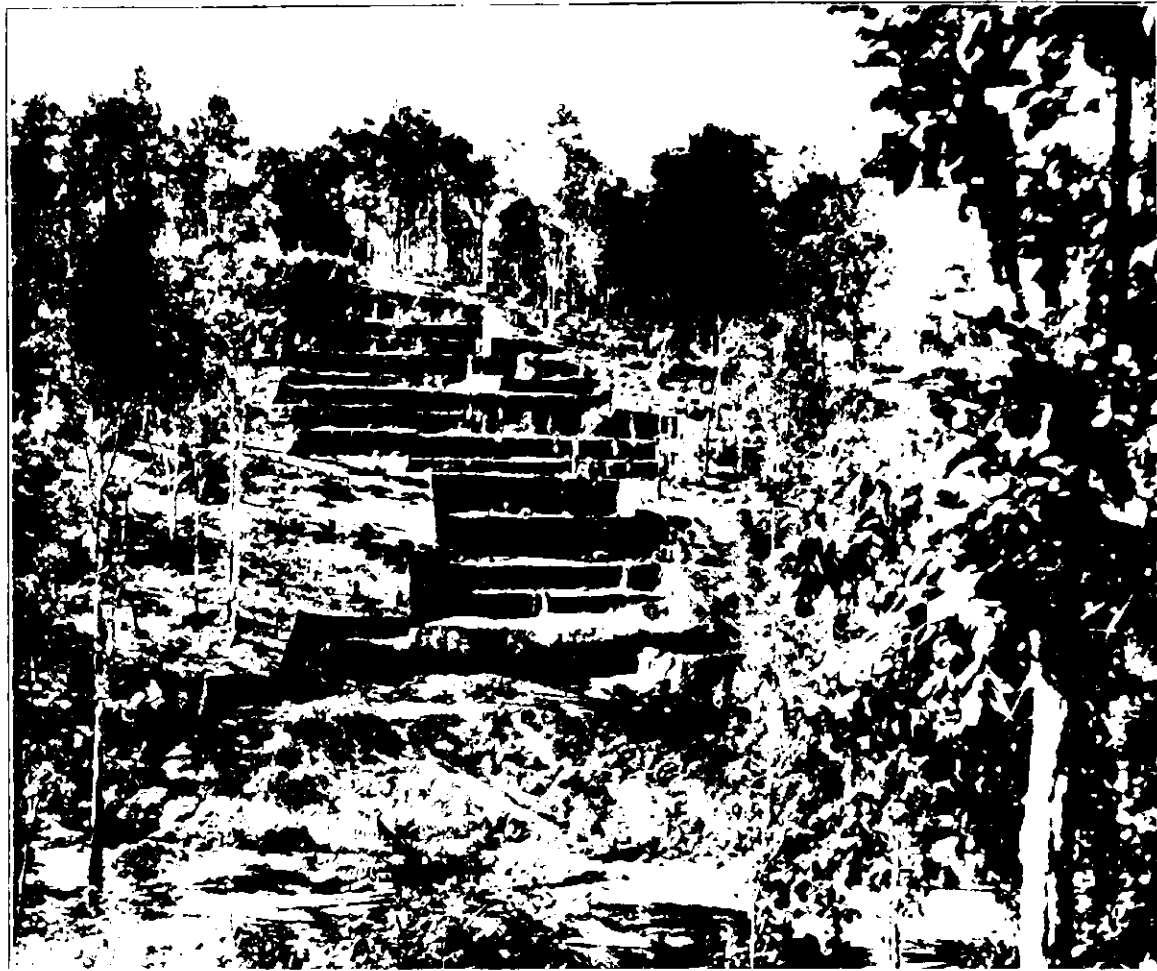
OPENING UP A MANGANESE ORE DEPOSIT
