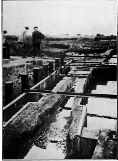
The view of the model after the bed and sides had been lined
