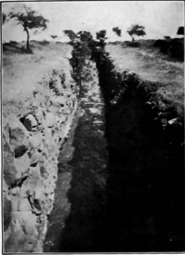
Malegaon Cut looking downstream when the present full-supply discharge of 452 cusecs was passing; showing the depth of the cut, roughness of the sides, etc.
