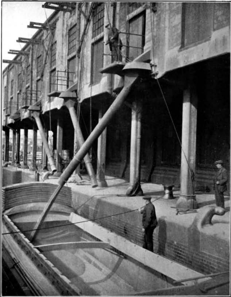
FIG. 14.—Barge being loaded with bulk grain ex elevator, Manchester.
