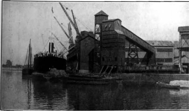
FIG. 21.—Liner discharging grain at Avonmouth, barges and a sailing vessel being loaded and sacked grain going to rail.
