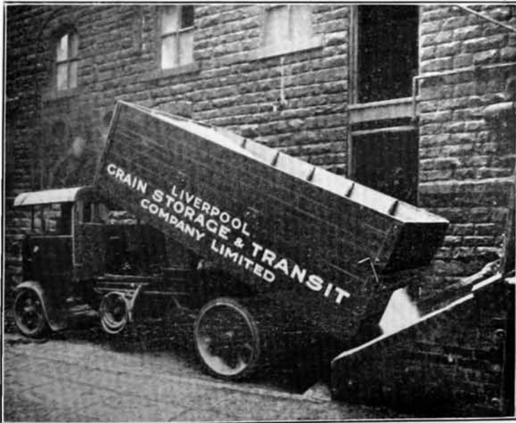
FIG. 30.—Unloading bulk grain from road wagon.
