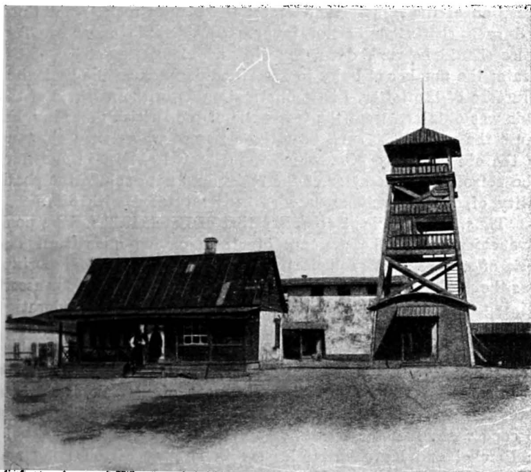
Fig. 4. Office at Berekei.
