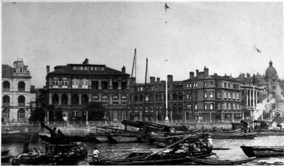
THE AMERICAN CONSULATE GENERAL AT SHANGHAI.—Typical of the buildings along the Bund, or Shanghai waterfront, of a few years ago, it suggests comparison with the new type of buildings on the Bund as represented by the home of the Hong Kong & Shanghai Banking Corporation in following picture.
