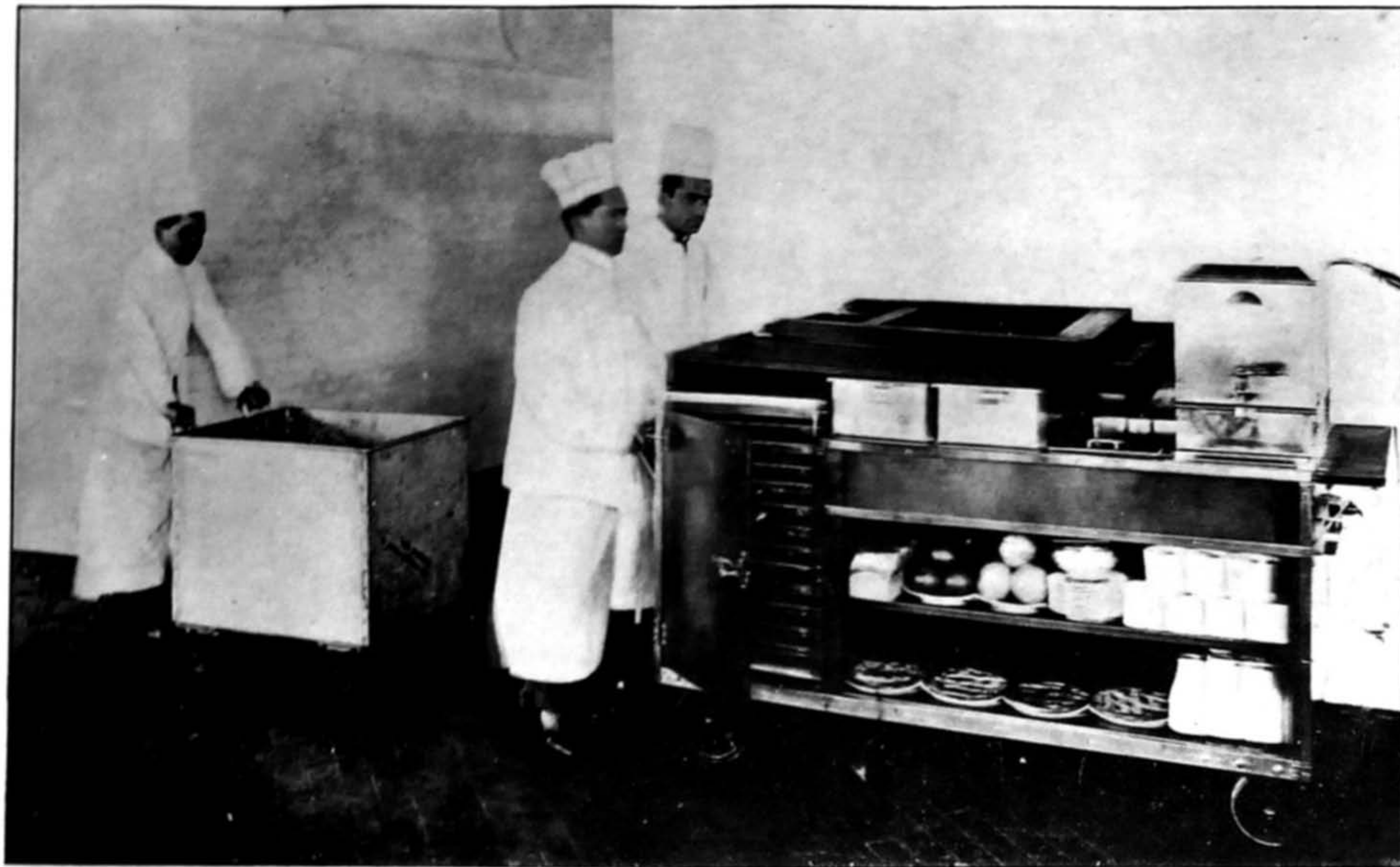
PLATE 19.—ELECTRICALLY HEATED CAFÉMOBILE EN ROUTE TO STATION IN PLANT.
