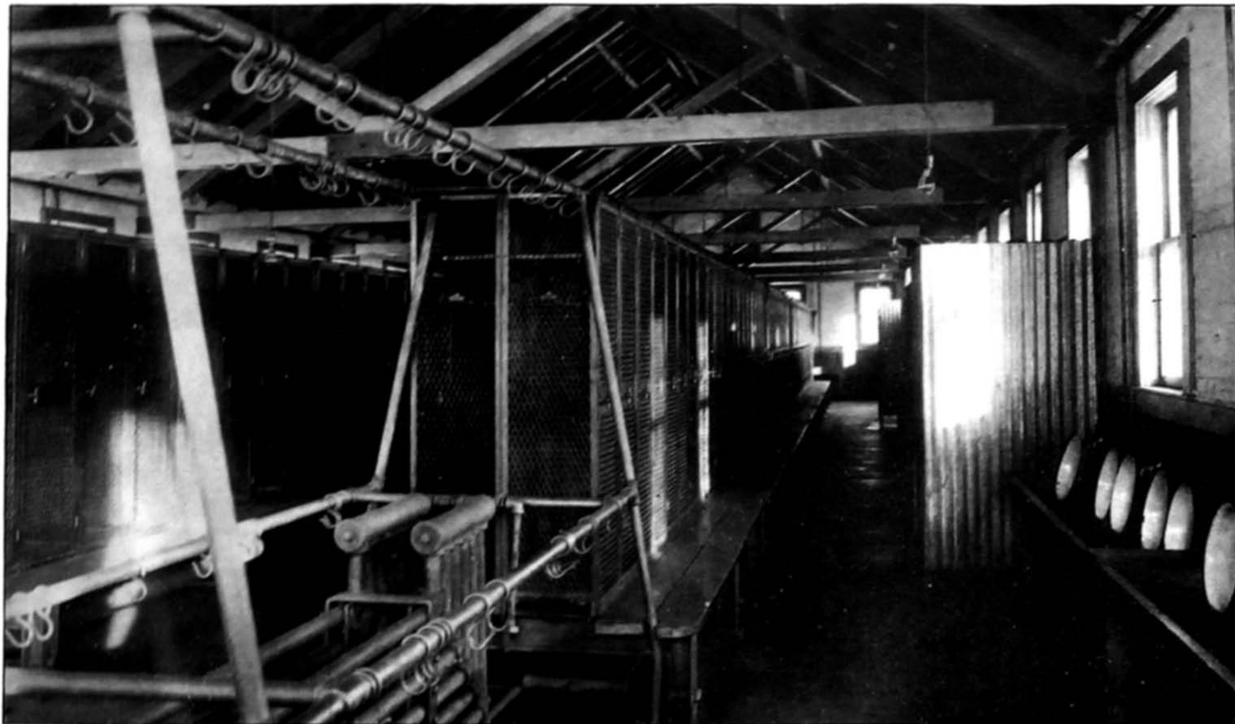
PLATE 15.—INTERIOR OF WASH AND CHANGE HOUSE; BASINS IN TROUGH, SHOWERS BEYOND; STEAM PIPES UNDER LOCKERS; BENCHES; S-SHAPED HOOKS ON STEAM PIPES FOR DRYING CLOTHING.
