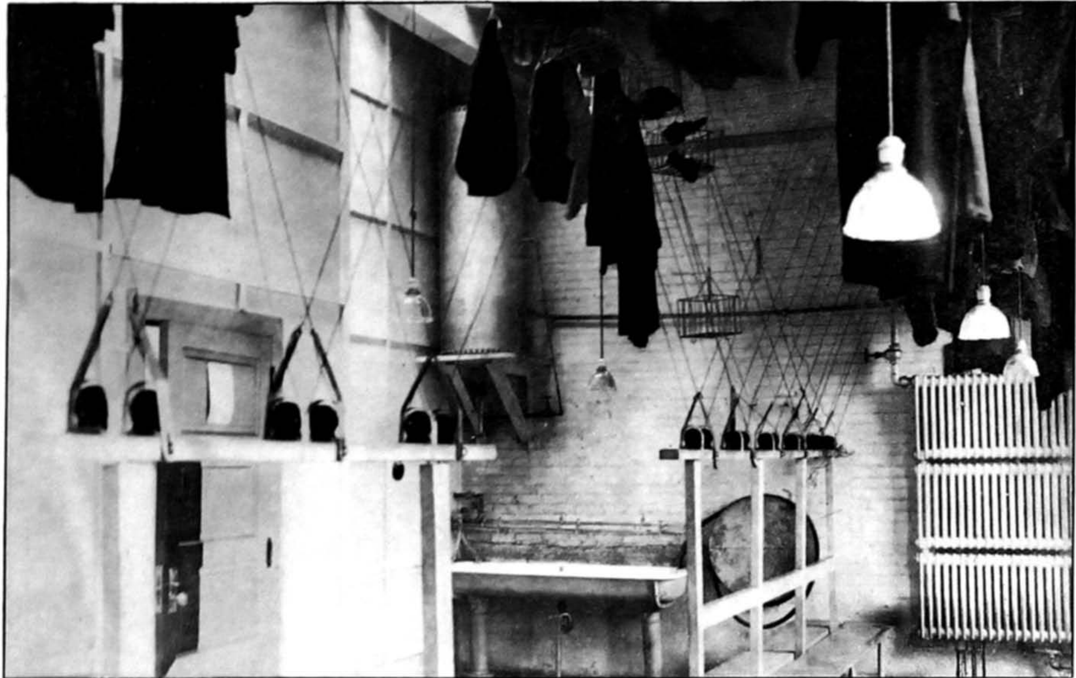
PLATE 17.—CHAIN LOCKERS, WHEREBY CLOTHES ARE RAISED TO ROOF AND FASTENED BY PADLOCK BELOW; RACKS FOR SMALLER ARTICLES, WITH HOOKS AT ENDS.
