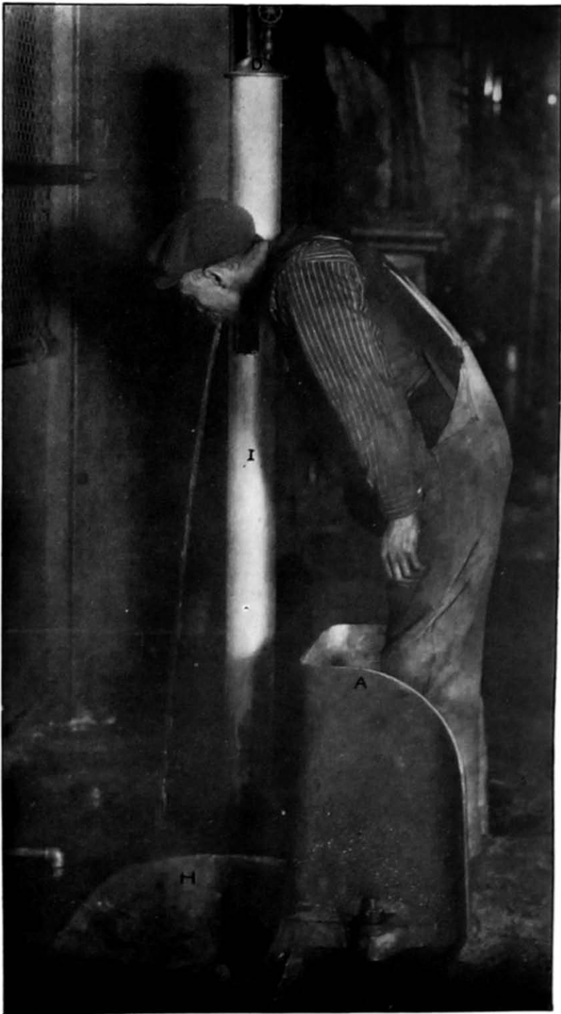
PLATE 12.—SANITARY DRINKING FOUNTAIN. SHOWING RELATION OF SPLASH GUARD "A" AND BASIN "H" TO POST "I."
