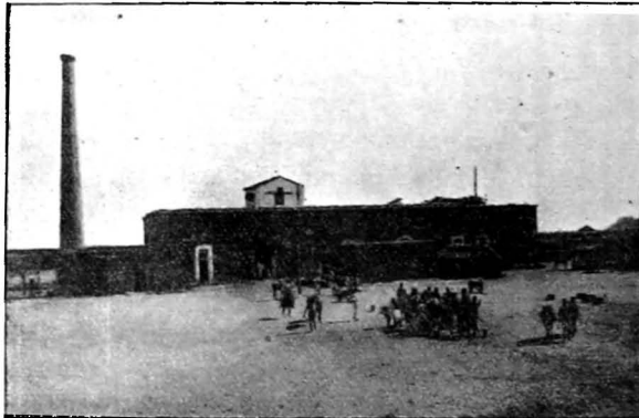
VIEW OF INTERIOR OF FORT KASSALA.
