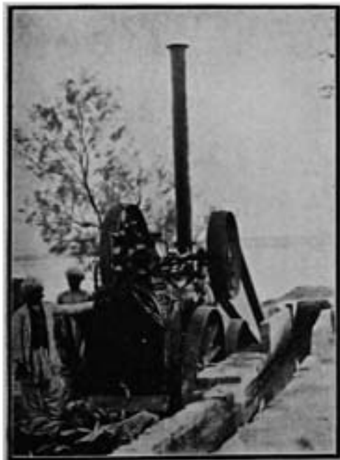
15. Pumping, by steam engine, direct from the River at Sukkur.
