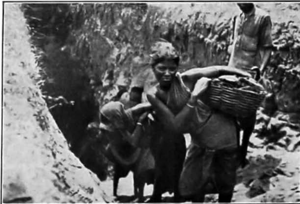
WOMEN WORKERS COMING TO THE SURFACE AFTER EMERGING FROM THE INCLINE SHOWN ABOVE. FROM THE INCLINE MOUTH THE COAL IS CARRIED UP A GRADIENT OF ABOUT 1 IN 2, FOR A DISTANCE OF 50 FEET. THE WOMEN ARE SEEN COMING UP THIS SLOPE.
