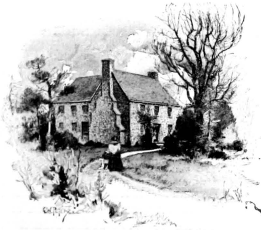
HOUSE AT GUILFORD, 1639
