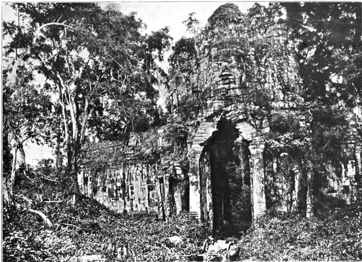
THE GATE OF VICTORY, ANGKOR-THOM
