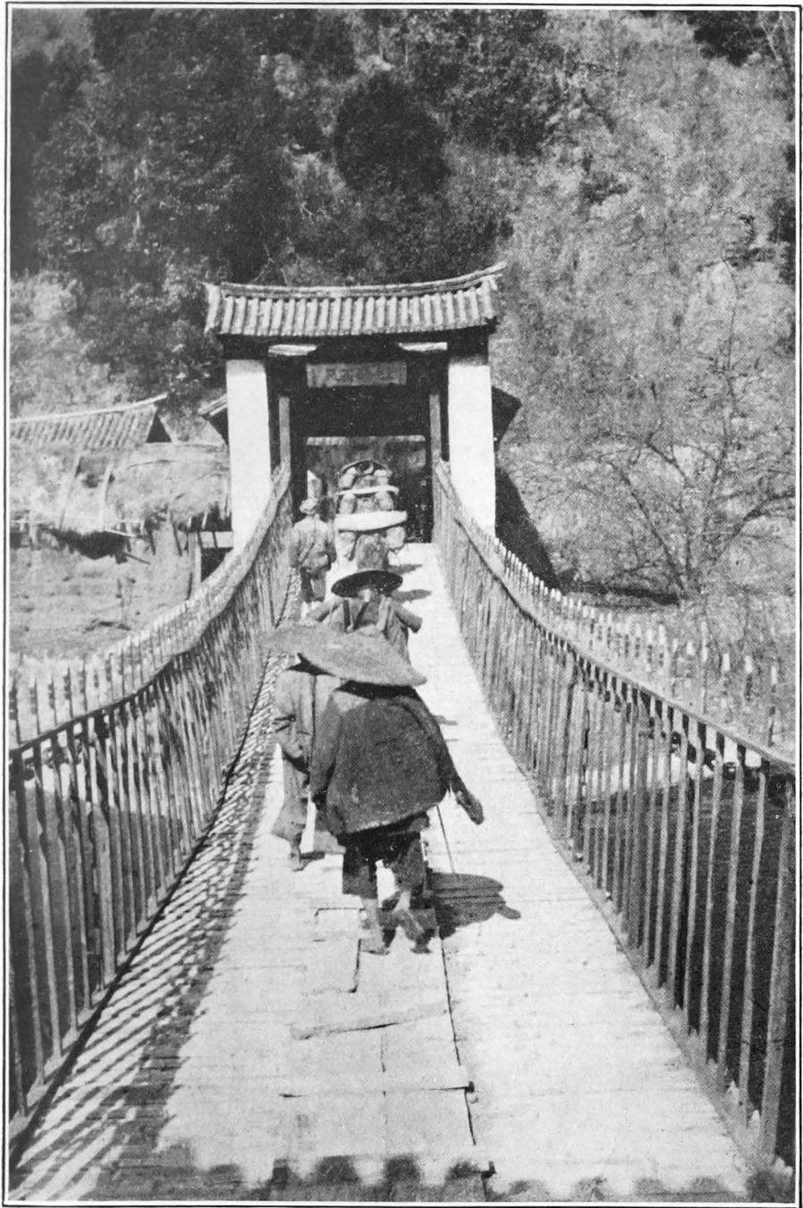
Bridge over the Mekong.
