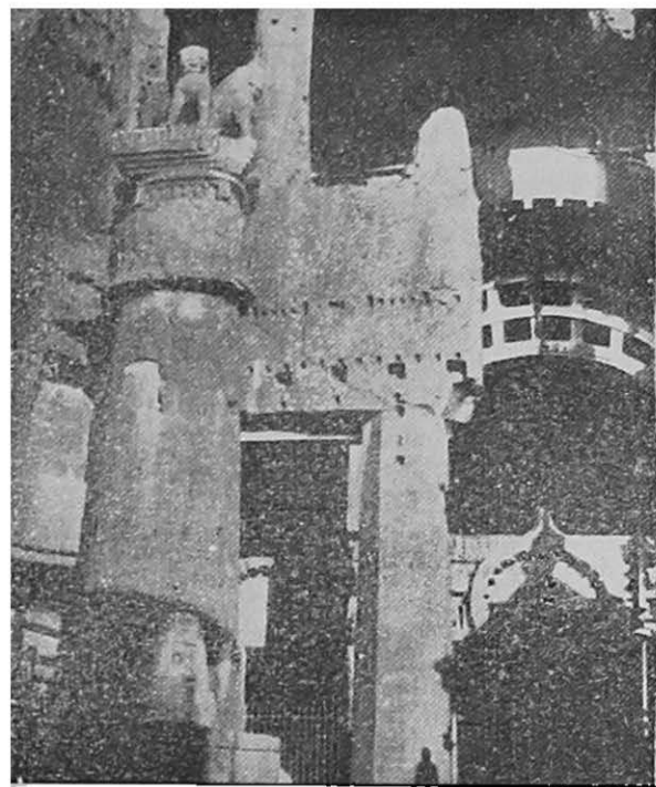
The Ashok Stambha at the entrance to the assembly hall (Karla Caves).
