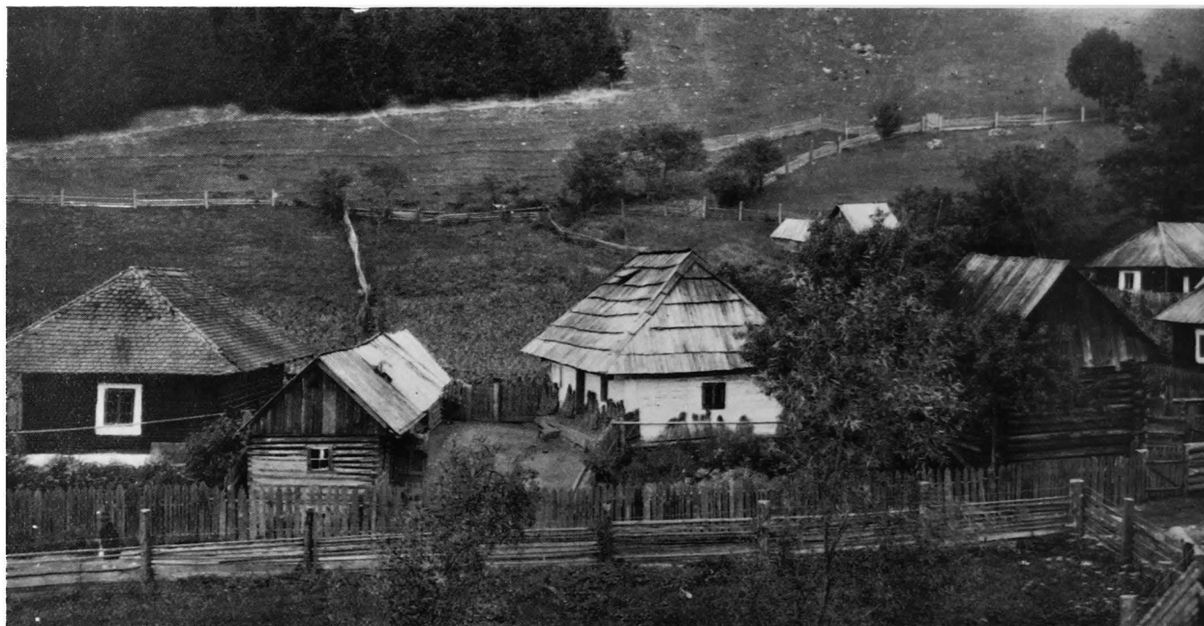
Typical Roumanian farmsteads in Corbu. The houses are roofed with shingles, the outbuildings with boards. The house in the centre has the characteristic louvre in place of chimney, and its walls are of timber with plaster covering. Hemp is drying on the verandah. The mud caulking in the outbuilding is clearly visible.
