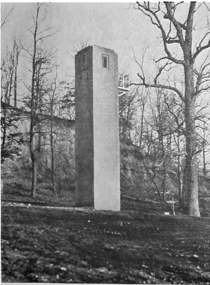
FIGURE 28.—Stream-gaging station on the Ohio River near dam 53. Special methods of stream-flow determination are necessary under flood conditions such as these.
