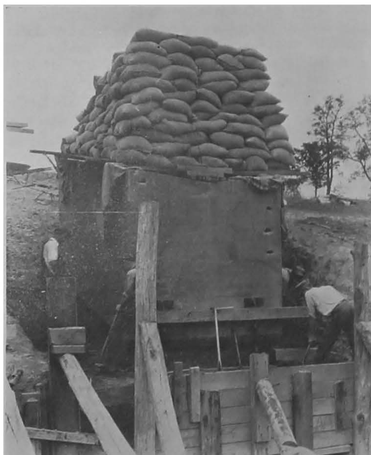
U. S. SOIL CONSERVATION SERVICE FIGURE 10.—The installation of a lysimeter at North Appalachian Experiment Watershed, Coshocton, Ohio. The lysimeter in the form of a bottomless box is heavily loaded with sand (10 tons in this instance) and the walls forced down around an undisturbed column of natural earth. The earth under the cutting edge is removed and the soil column carefully shaped to fit the interior of the lysimeter.
