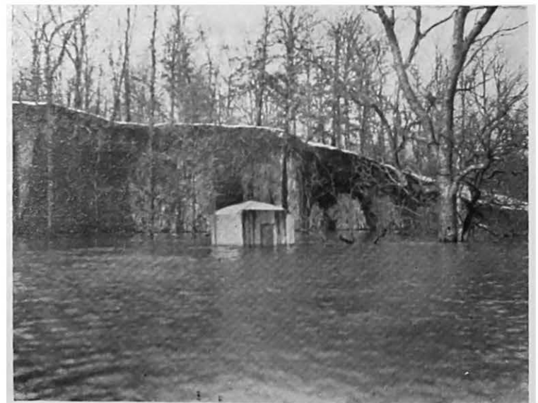
FIGURE 28.—Stream-gaging station on the Ohio River near dam 53. Special methods of stream-flow determination are necessary under flood conditions such as these.
