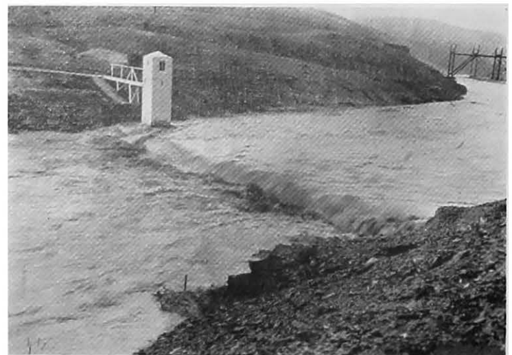
FIGURE 24.—Two views of the gaging station operated by the Geological Survey on Duck Creek in the Copper Basin area of Tennessee. Smelter fumes have completely denuded the area of vegetation resulting in a rapid run-off and heavy erosion. The discharge shown occurred within one hour after a moderate rainfall over the 13.0 square mile watershed. A maximum run-off of 7,080 second-feet (545 c. f. s./s q. mi.) was recorded on April 6, 1936.
