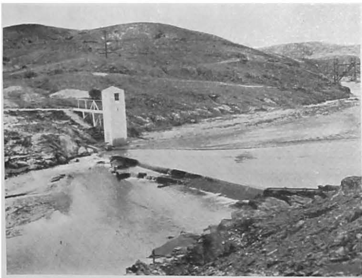
FIGURE 24.—Two views of the gaging station operated by the Geological Survey on Duck Creek in the Copper Basin area of Tennessee. Smelter fumes have completely denuded the area of vegetation resulting in a rapid run-off and heavy erosion. The discharge shown occurred within one hour after a moderate rainfall over the 13.0 square mile watershed. A maximum run-off of 7,080 second-feet (545 c. f. s./s q. mi.) was recorded on April 6, 1936.
