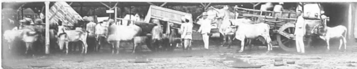
CAMP EQUIPMENT BEING LOADED INTO STORE GODOWNS.
