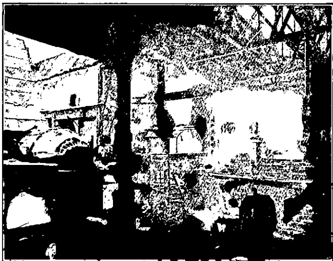
BESSEMER CONVERTER AT EDGAR THOMSON WORKS, PITTSBURG
