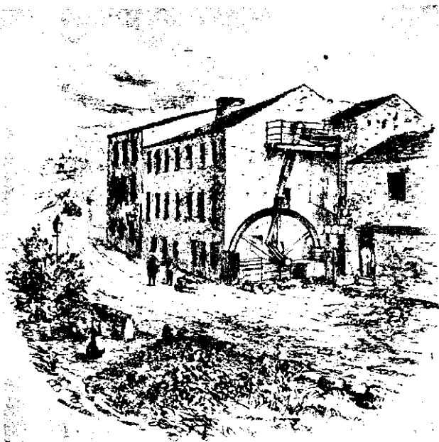
CRANK MILL, Morley, Yorkshire. Built in 1790, this mill was driven by steam and was the first to be erected in the neighbourhood.
