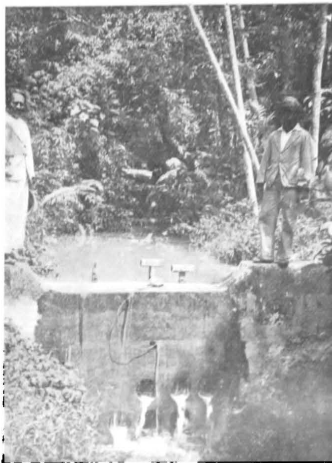
Figure 6. —Anti-larva sluicing in Malaya. One type of dam with hand-operated release.
