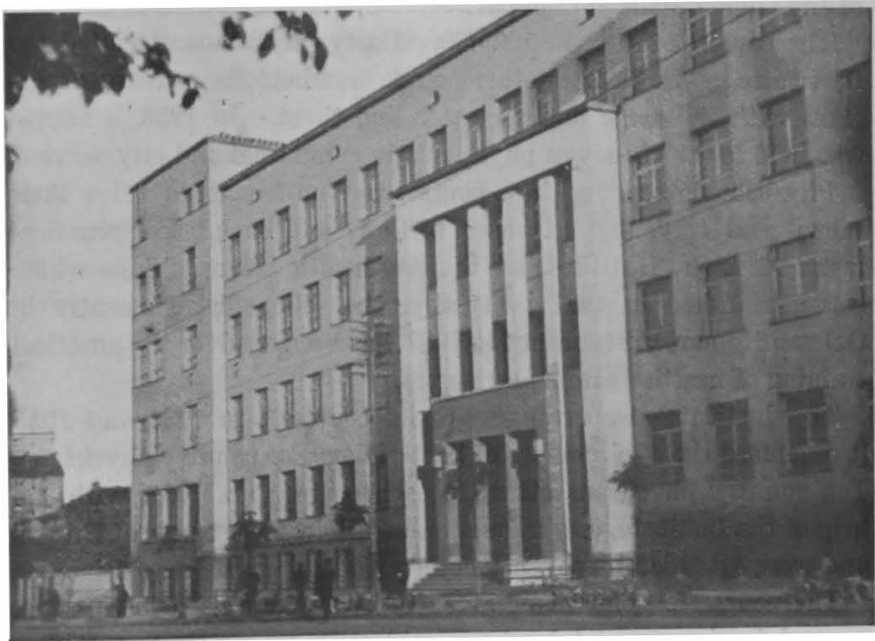
Figure 13. —FRONT VIEW OF THE INSTITUTE OF PUBLIC HEALTH AT SOFIA.
