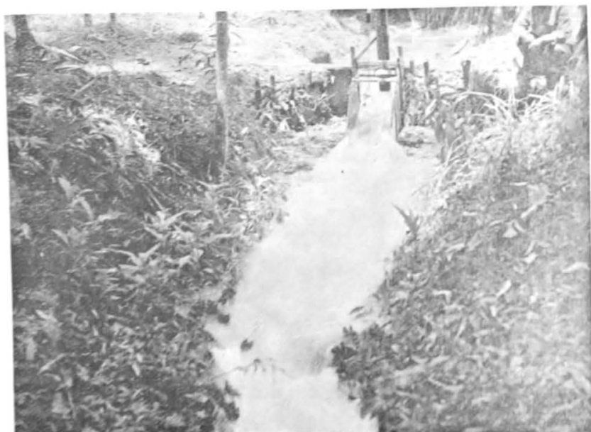
Figure 10. —The jigger shown in Figure 9 automatically discharging a reservoir estimated to contain about 15,000 gallons of water. (Courtesy of K. B. Williamson.)
