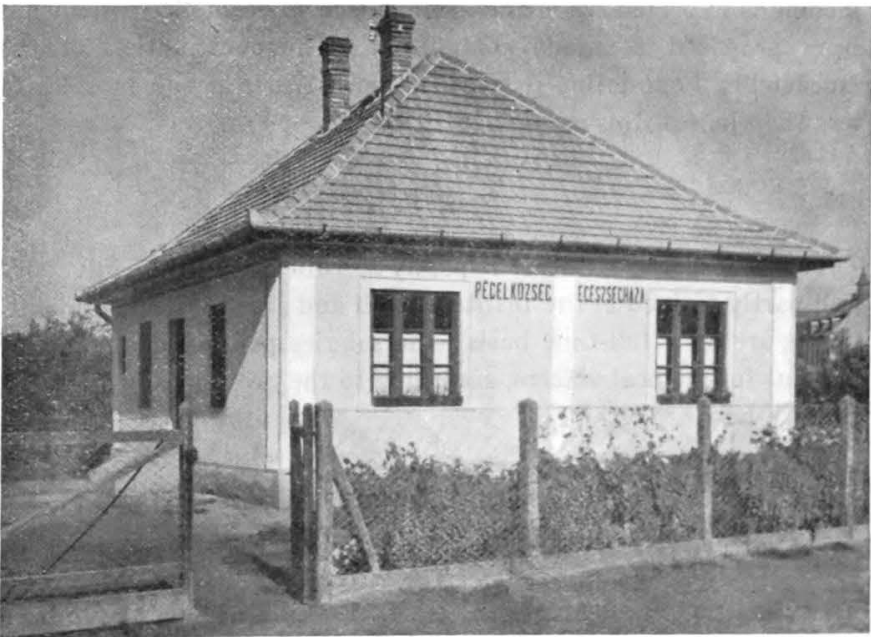
Figure 6. —HEALTH CENTRE AT PÉCEL.
