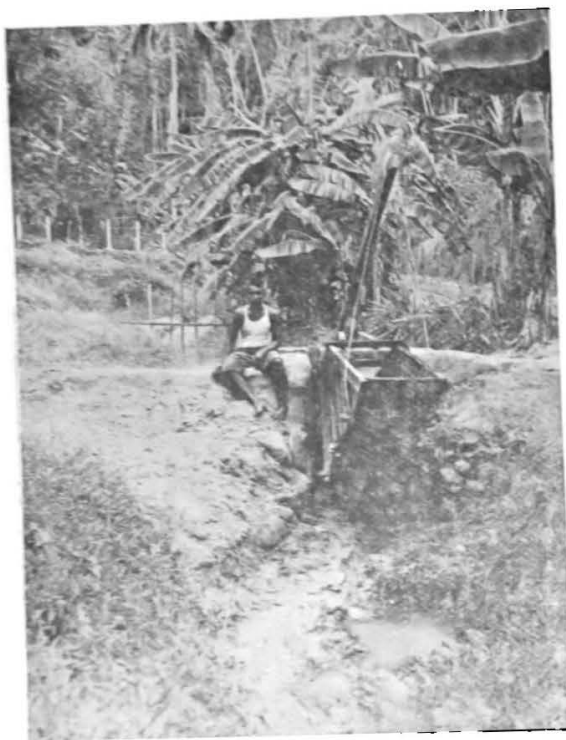
Figure 9. —A similar jigger set in concrete about to discharge the reservoir into a flat grassy channel. (Courtesy of K. B. Williamson.)
