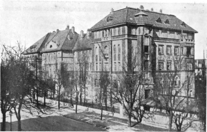
Figure 5. —STATE INSTITUTE OF HYGIENE AT BUDAPEST : MAIN BUILDING.
