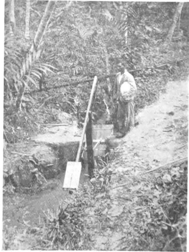
Figure 8. —Williamson's automatic tipping sluic-gate or "jigger", with counterbalancing weight, seen from up-stream, awaiting discharge when water level rises. (Courtesy of K. B. Williamson.)
