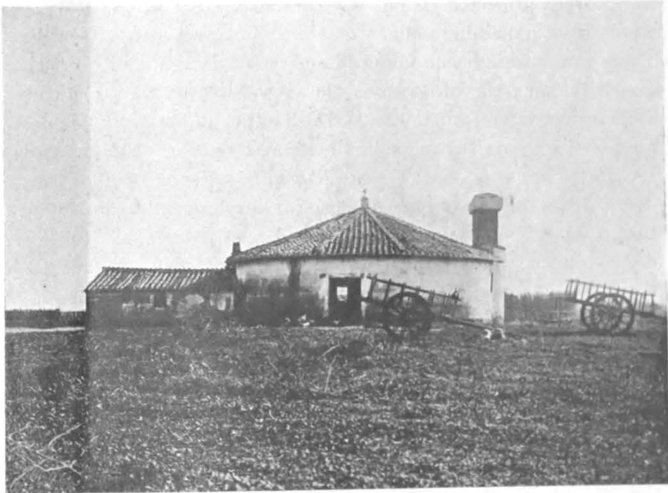
Fig. 2. — TYPICAL FARM BUILDING AT THE FOOT OF THE MOUNTAIN.
