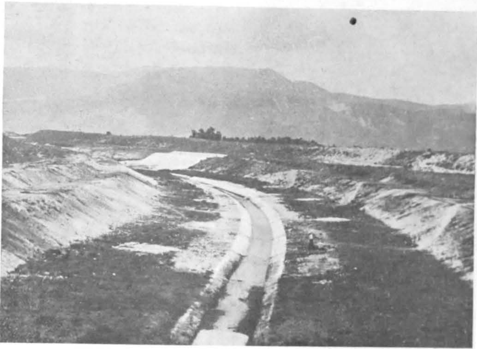
Fig. 11. — THE MUSSOLINI CANAL UNDER CONSTRUCTION, WITH ITS CENTRAL RUNNEL.
