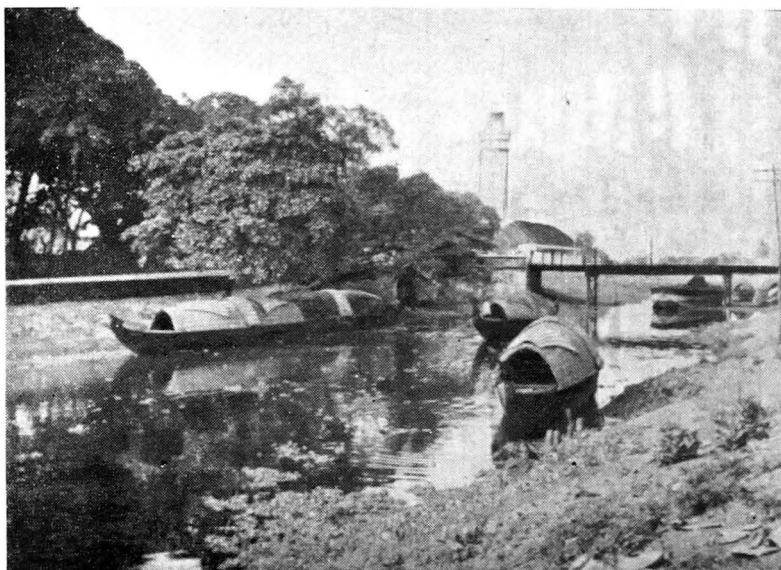
Neglected state of a canal in Alleppey.
