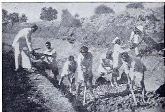
Levelling the road.
