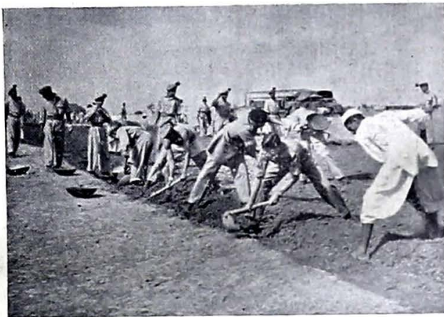
(d) Social service work by Cadets. A road being constructed.
