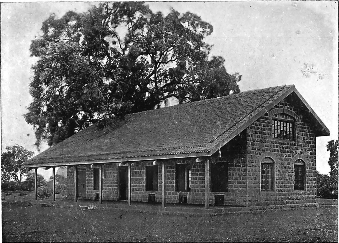
LOCAL BOARD PRIMARY SCHOOL, NIMBGAONJALI, TALUKA SANGAMNER, AHMEDNAGAR DISTRICT (BOMBAY).
