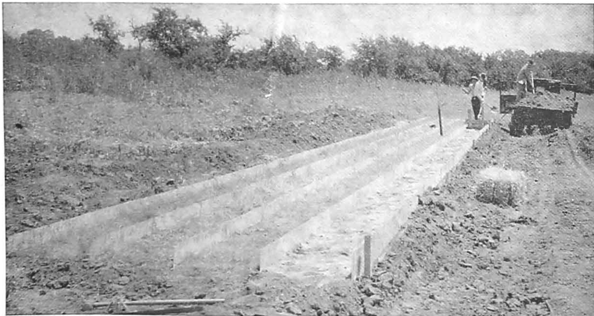
Fig. 3.—Installing sheet iron separators between channels. Strips of sheet iron 18 inches wide were placed 12 inches below finished grade and 6 inches above. Note 2" x 12" boards used for maintaining alignment while soil is placed in channel.
