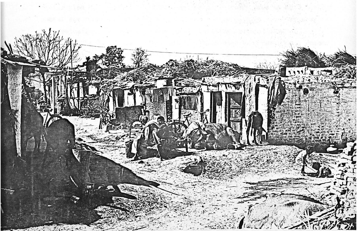
11. (Above) One and a half room tenements in double storeyed blocks under construction for resettlement of some 'labour colony' residents. 12. (Below) A street and use of space in one of the 'labour colonies'.
