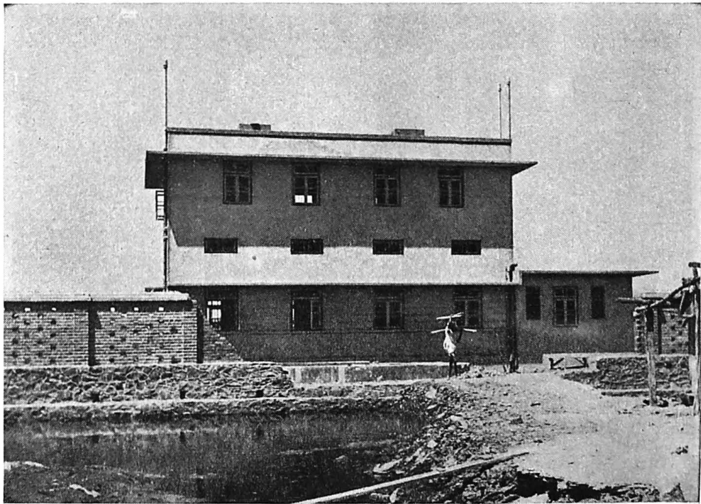
Kurla pumping station
