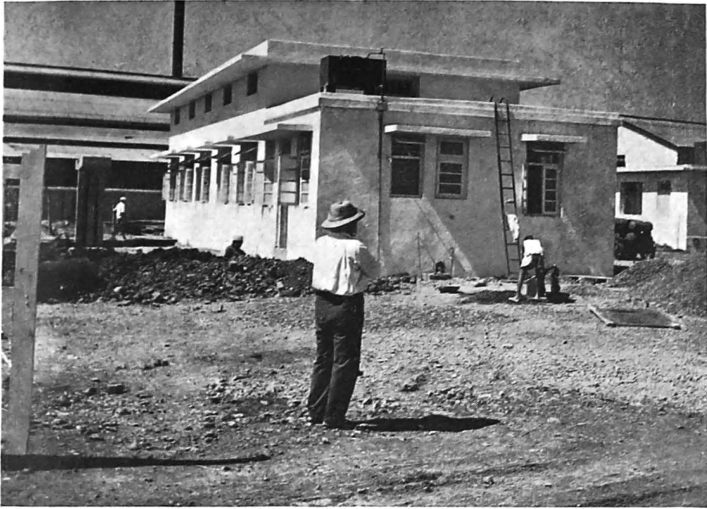
Ghatkopar pumping station
