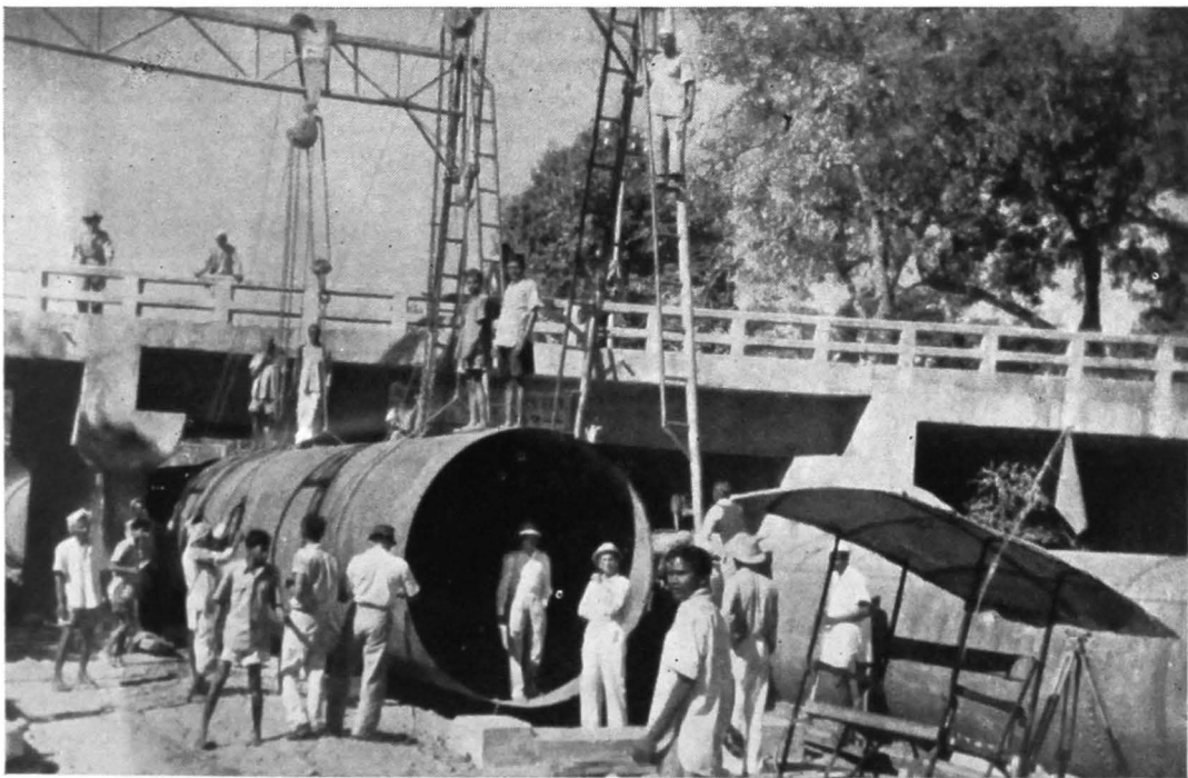
96" Dia. Pipe Line being laid Under an Over bridge Near Kapurbawdi
