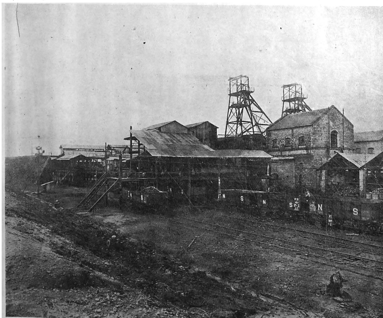
Coal Screening Plant, Singareni.
