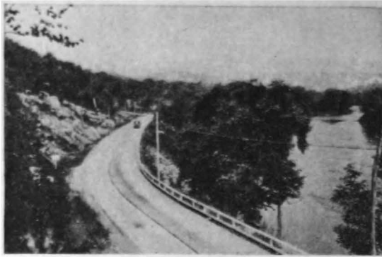
A SECTION OF THE HOUSATONIC RIVER ROAD NORTH OF NEW MILFORD IMPROVED WITH CONCRETE
