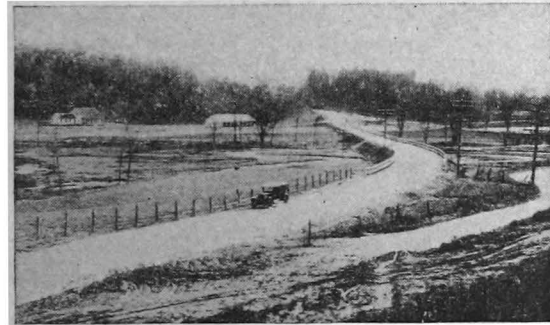
A SECTION OF THE KENT-MACEDONIA ROAD, TRUNK LINE NO. 127, SURFACED WITH WATERBOUND MACADAM. (THE OLD LOCATION IS SHOWN AT THE RIGHT)
