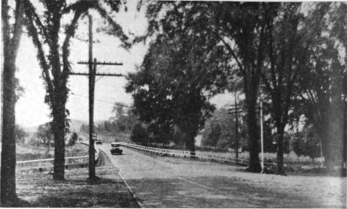
A SECTION OF THE NORWALK-DANBURY ROAD LOOKING SOUTH AT KELLOGG'S CORNER
