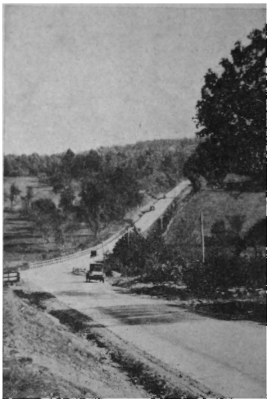
THE OLD ROADS FOLLOWED IN MANY CASES THE LINES OF ANCIENT TURNPIKES; AND NOT ENOUGH ATTENTION HAS BEEN GIVEN TO THE CORRECTION OF ALIGNMENT WHEN THESE ROADS HAVE BEEN RECONSTRUCTED
