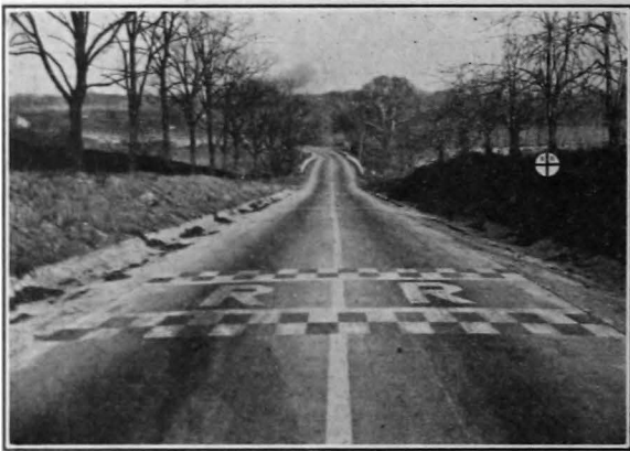
Surface Marking on the Highway Indicating the Approach to a Railroad Grade Crossing Near Hummelstown.
