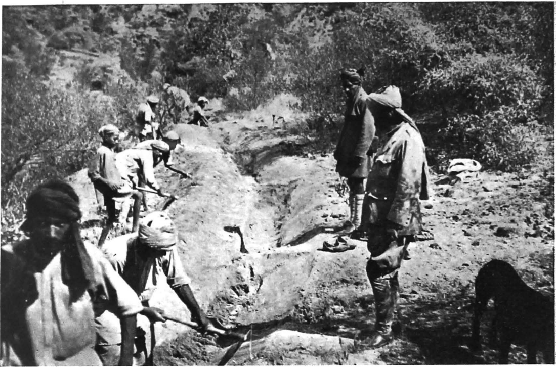
An open type of contour trench which has given good results in water-catching and encouragement of vegetation. Dimensions :—
