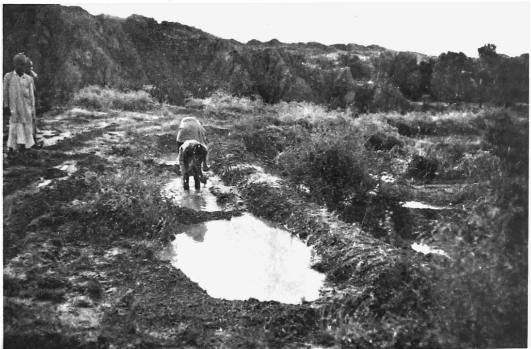
A good catch of rain in the contour trenches continues to seep into the ground for several days after the storm and long after untrenched slopes are again bone-dry.
