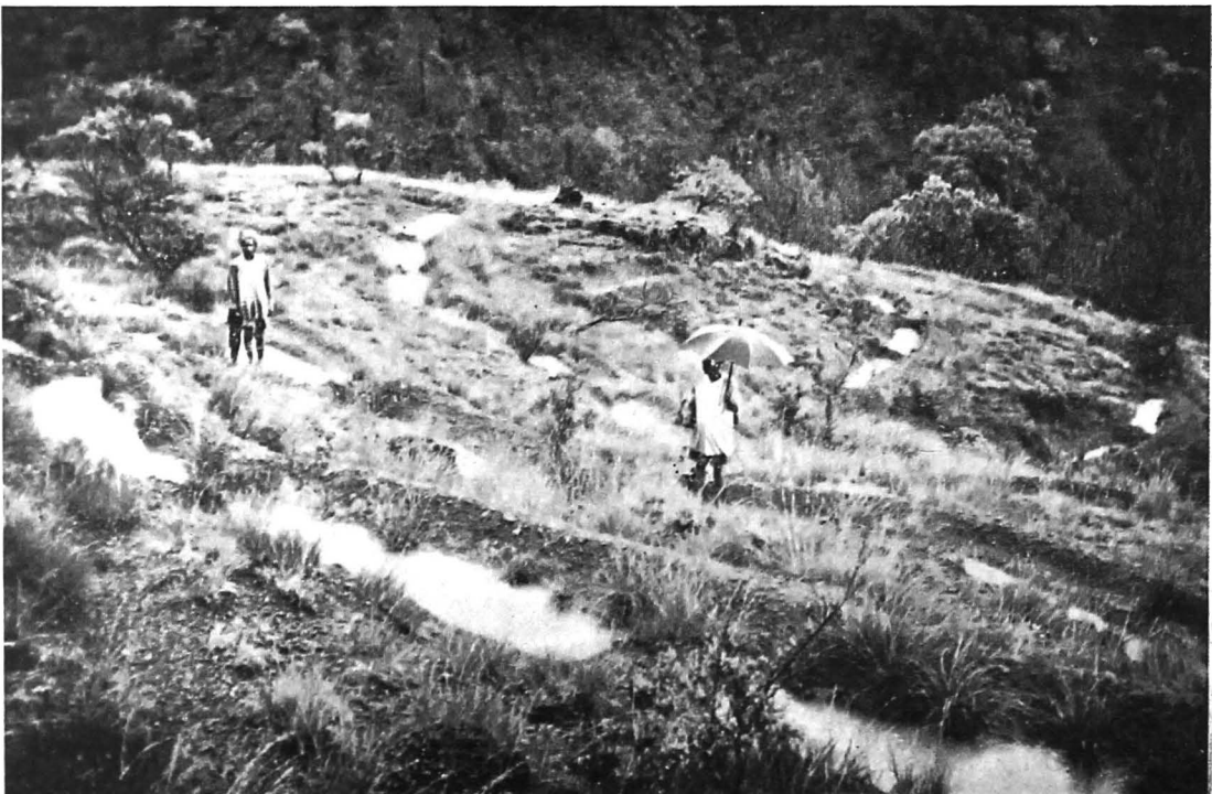
Contour trenches at Dholbaha in head of Paphial Cho, with their first catch of rain water. Planted bhabbar grass cannot be seen but vestiges of original anjan and daulu grasses are already profiting by moisture.
